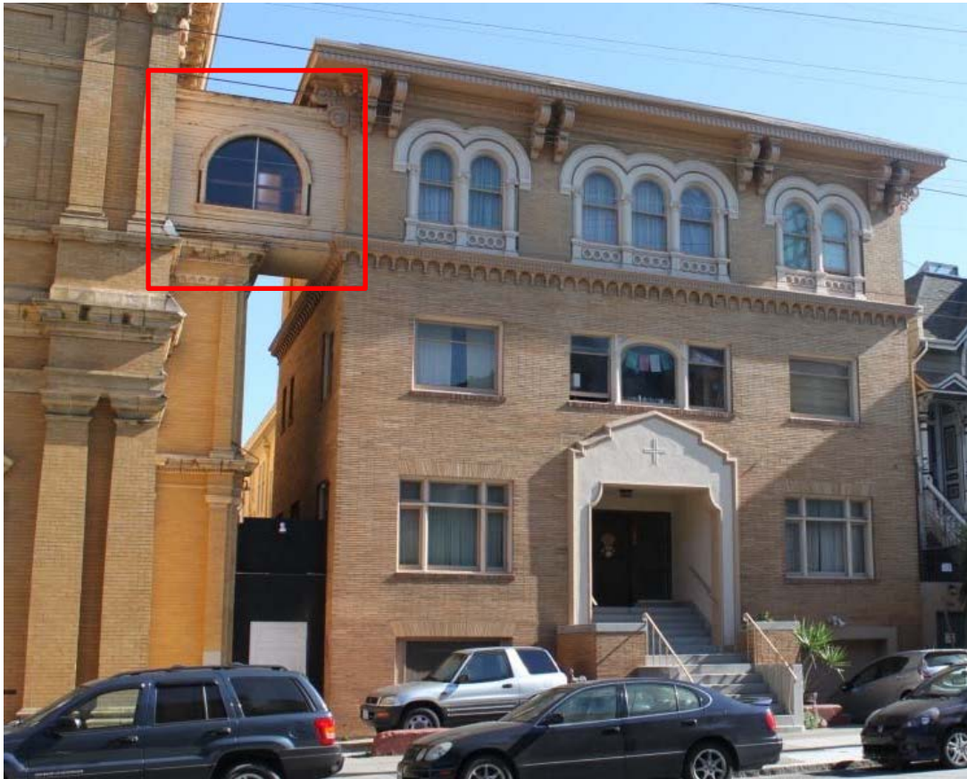
Photo 1. Exterior view of connector (outlined in red) between the third story of the rectory and the choir loft, view east, 2016. It was constructed sometime between 1913 and 1920 to allow priests easy access to the sanctuary for early morning masses and to get between the church and rectory in inclement weather.
