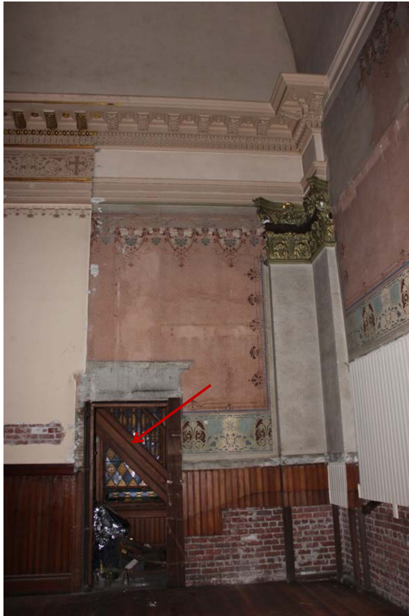
Photo 3. Choir loft, view south, 2016. Note the opening and stair (indicated by red arrow) that leads to the connector. The pipe organ was installed in 1923 and it blocked access to the connector. When the organ was removed sometime after 2009, the opening to the connector, as well as decorative wall painting dating from an earlier period was exposed. Also note ghosting above the opening from trim that was likely removed to install the organ.
