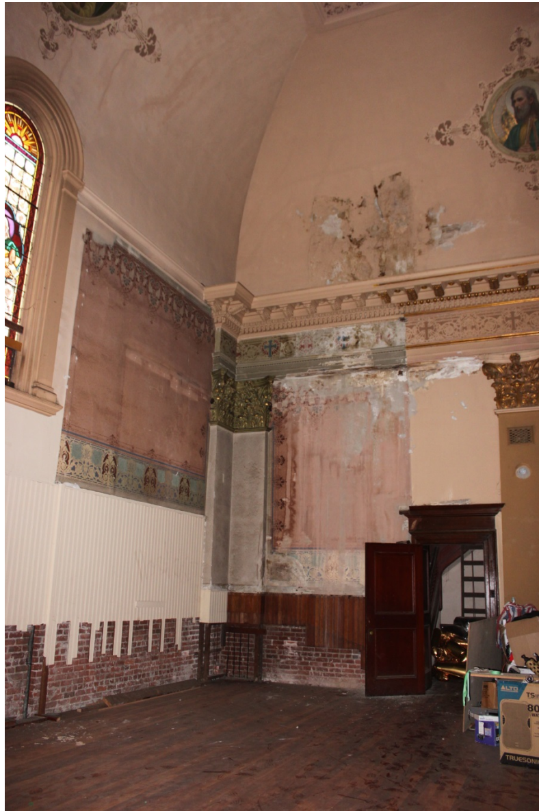
Photo 4. Choir loft, view northwest, 2016. Note decorative wall painting dating from an earlier period that was exposed when the organ was removed. Opening at right provides access to campanile stair. Trim above opening is likely similar to the trim that was removed at the connector opening to install the organ in 1923.
