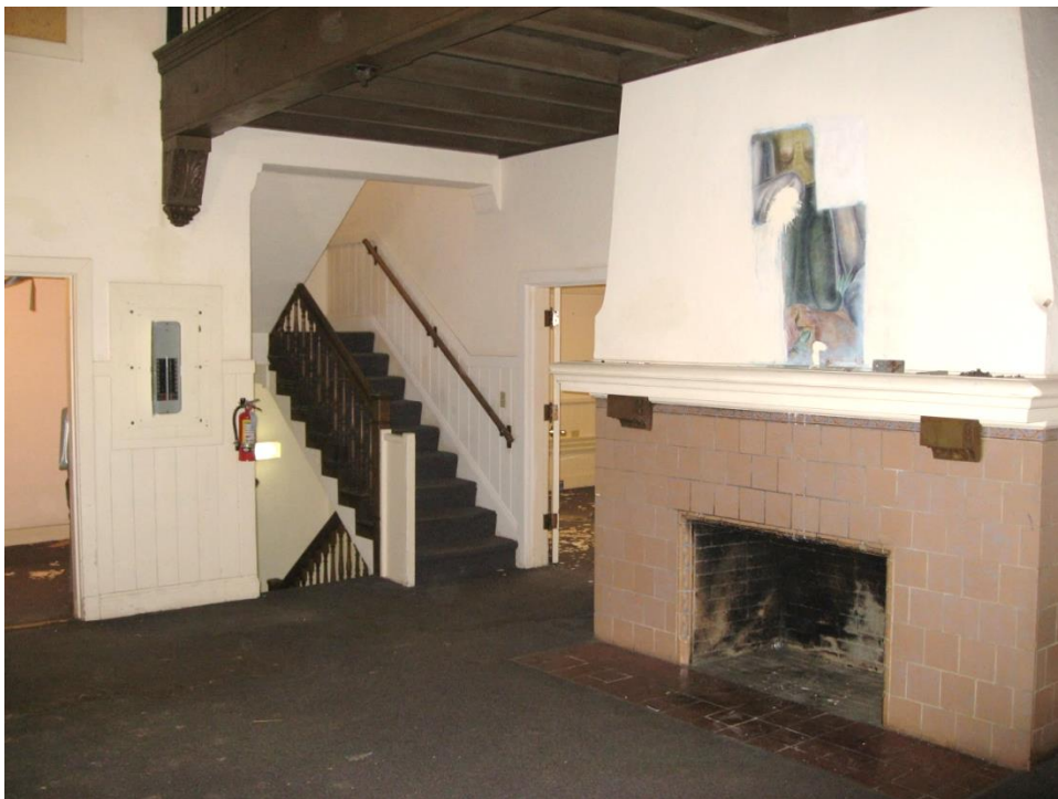
Detail of staircase and fireplace; on fireplace note tile cladding, wood brackets supporting mantle and over-painted fresco above.
