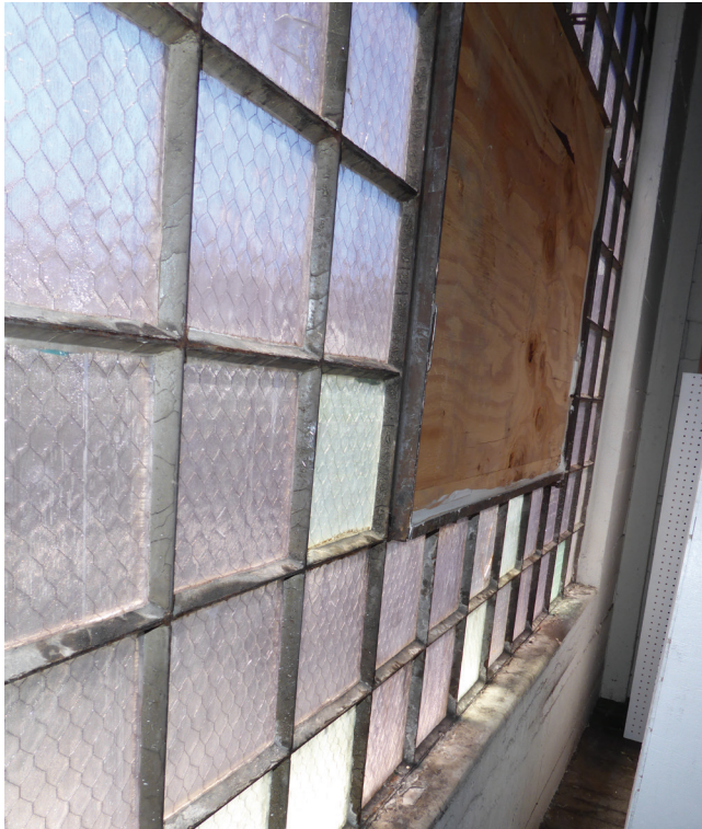
(Window 3.4) Typical overall condition of third story windows, with plywood infill at the hopper.
