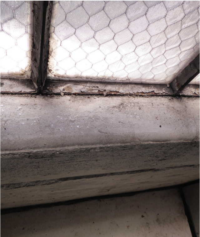
Typical condition: Failing putty and minor corrosion at sill.
