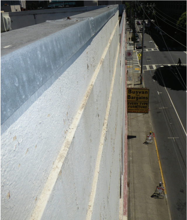
3. Typical condition (good) of parapet and parapet cap.
