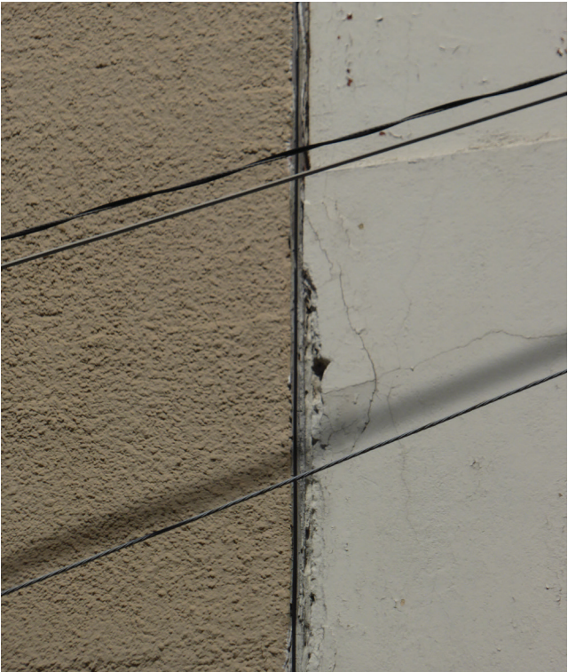
4. Spalling, bursting, and cracking at party wall with 950 Battery Street.
