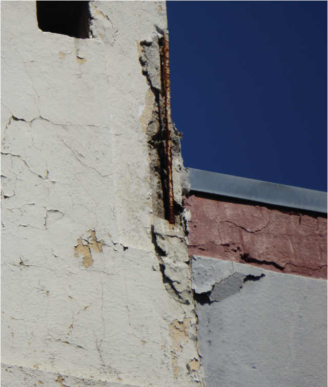
1. Spalling and bursting associated with the corrosion of the steel reinforcing.
