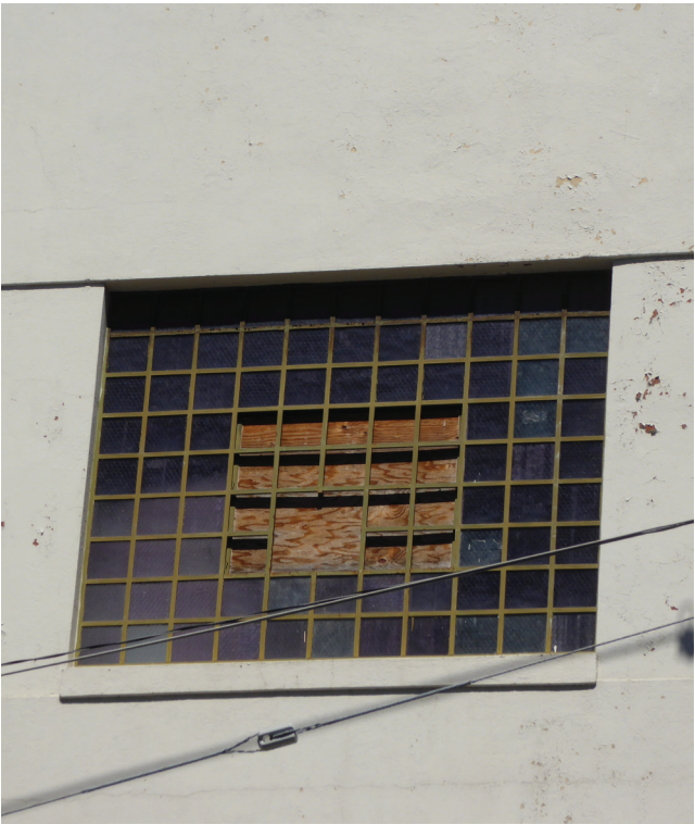
(Window 3.4) A small section of the historic muntin grid has been cut out near the bottom of the historic hopper location.
