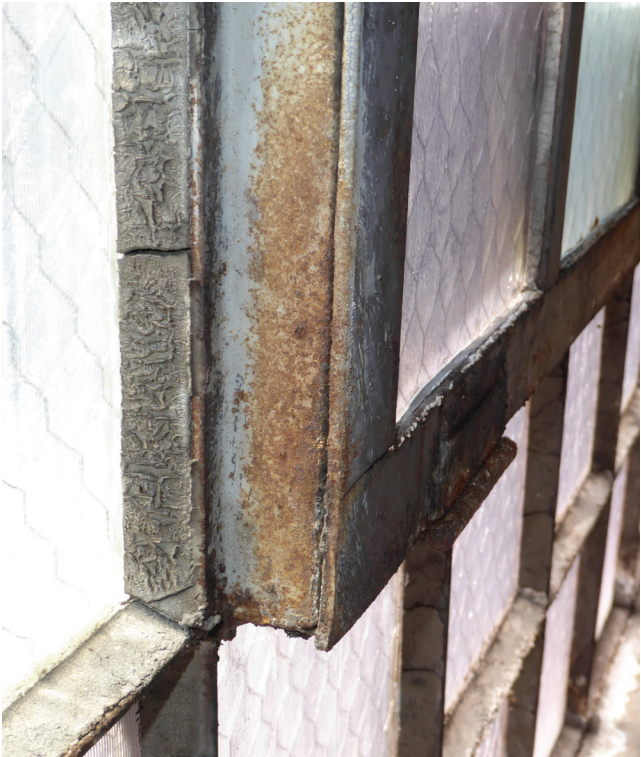
(Window 3.1) Failing putty, and minor surface corrosion at hopper.
