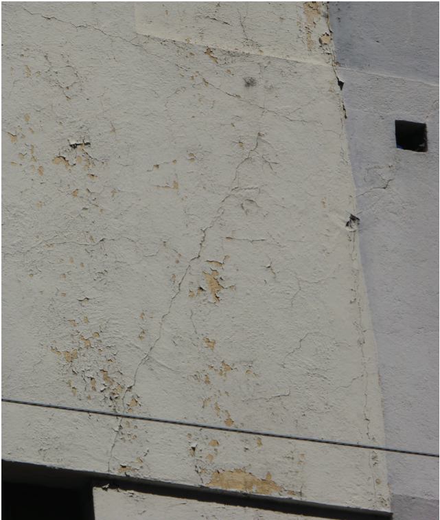
6. Shear cracking and map cracking in the cement plaster.
