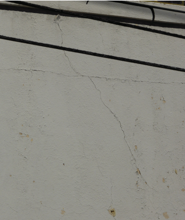
5. Typical shear cracking.
