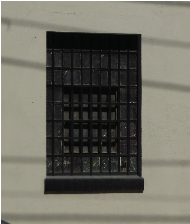
(Window 1.1) Condition of paint coatings is better than at the third story, and there appears to be less corrosion as a result.
