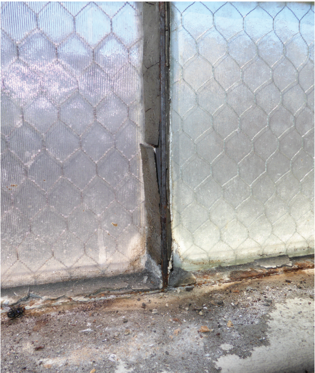
(Window 3.2) Failing putty and evidence of water intrusion at sill.
