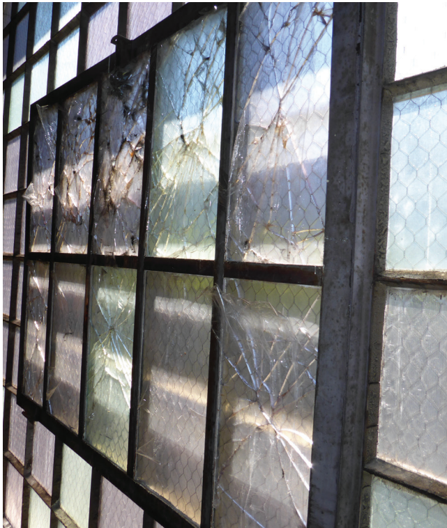
(Window 3.3) Extensive damage to glazing in hopper section.
