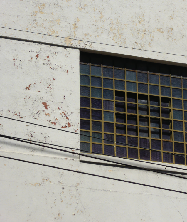
2. Typical condition (fair)-failing paint over cement plaster.
