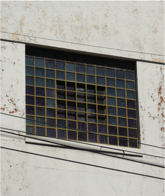
(Window 3.1) Typical conditions of all third-story windows: failing paint coatings and surface corrosion present. Corrosion appears to be worse near the window head.
