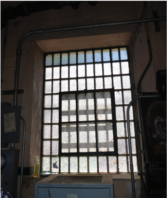
(Window 1.1) Overall condition - extensive damage to glazing.
