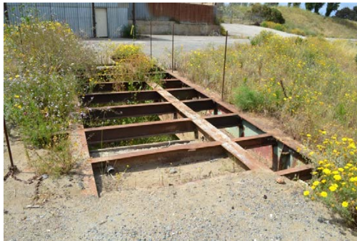
Figure 62. Exposed steel road undergirding, viewed facing northwest
