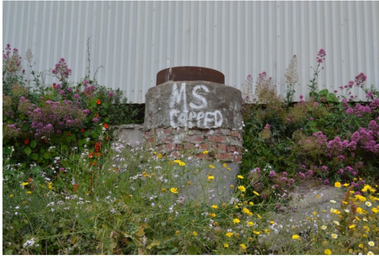
Figure 65. Sewer standpipe, viewed facing northwest
