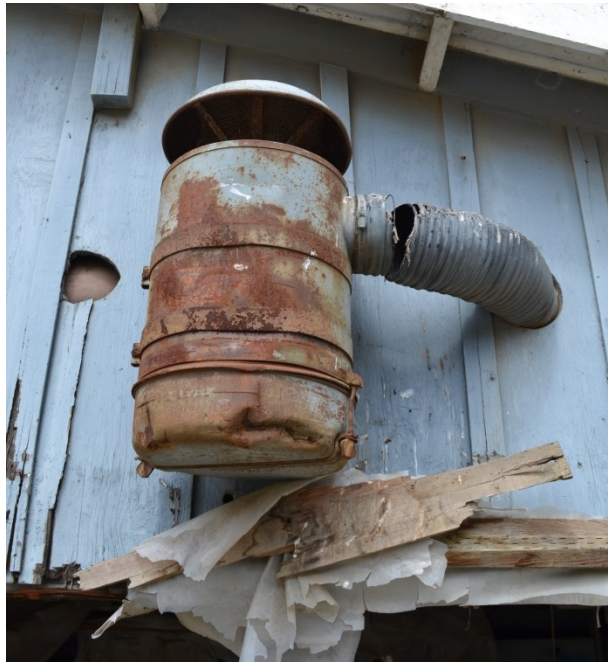
Figure 46. Detail of mounted ventilator
