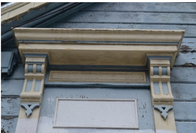
Figure 6. Window transom panel and architrave detail
