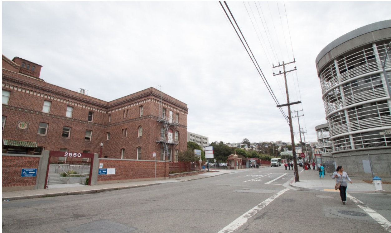
Figure 3. View of Building 9 and B/C Lot, looking east (Architectural Resources Group, August 4, 2015).
