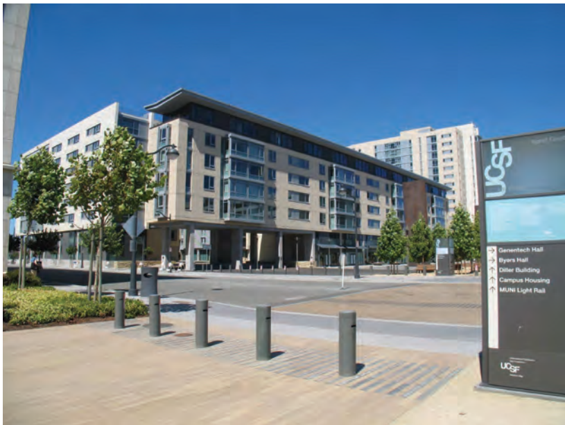
Guideline 2: A major crossing of Fourth Street at Mission Bay has been improved with special paving and bollards.
