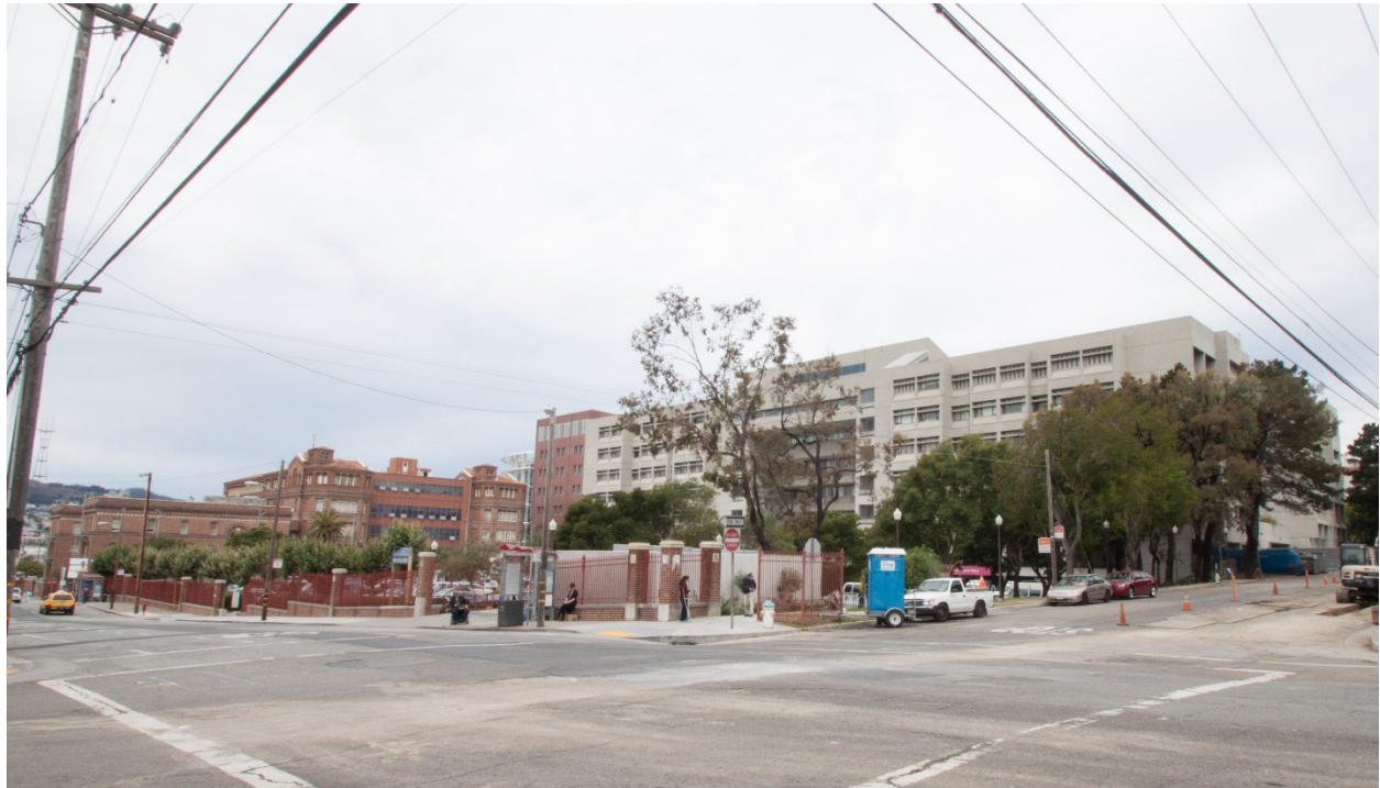
Figure 1. View looking northwest of B/C Lot (Architectural Resources Group, August 4, 2015).
