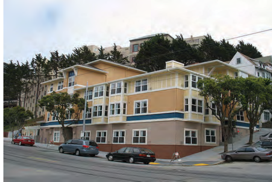
Guideline 3a: This campus residence at Parnassus Heights relates to the residential architectural vocabulary of the surrounding neighborhood.
