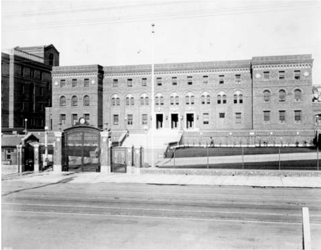
FRONTAL VIEW OF BLDG. 25 (DEMOLISHED)
