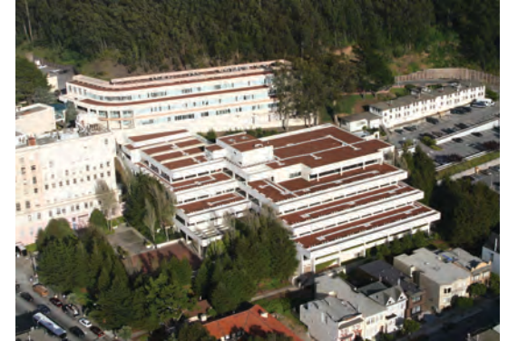
Guideline 3b: The Dental Clinics building steps down on its site serving to reduce its apparent mass and bulk.
