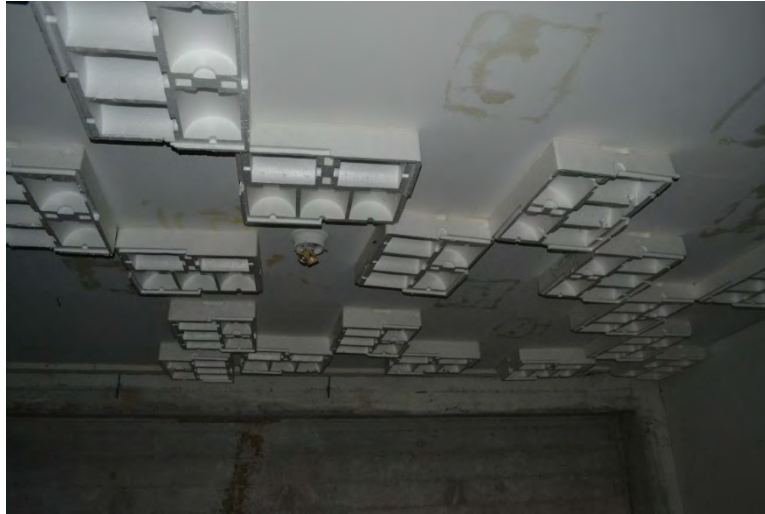
Figure 31. 665 Harrison Street, acoustic ceiling pads
