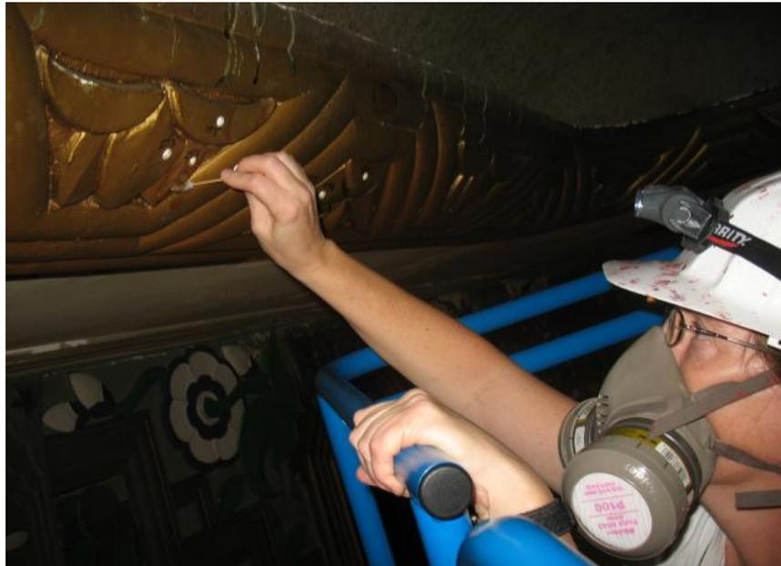
Sample methodologies: applying chemical solvents (above) and procuring samples for microscopic analysis (below).
