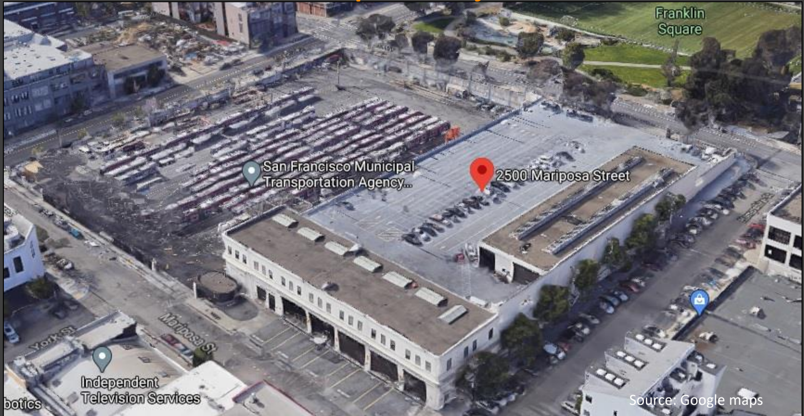
Oblique aerial view of project site showing 2-story office wing along Mariposa Street and rear maintenance wing along Hampshire Street
