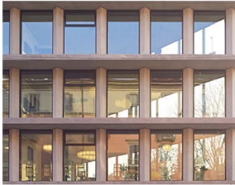
Low-iron glass windows Upper volume facade & lower volume windows (image from HdM's Feltrinelli)
