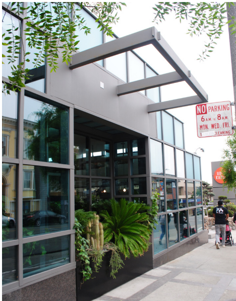
Landscape elements can help buffer the transition zones between inside and outside.
