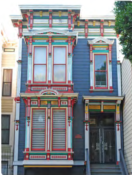
Victorian buildings provide an opportunity for vibrant facade expressions.
