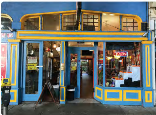
French doors in place of storefront windows creates an easy transition from the business to the sidewalk.
