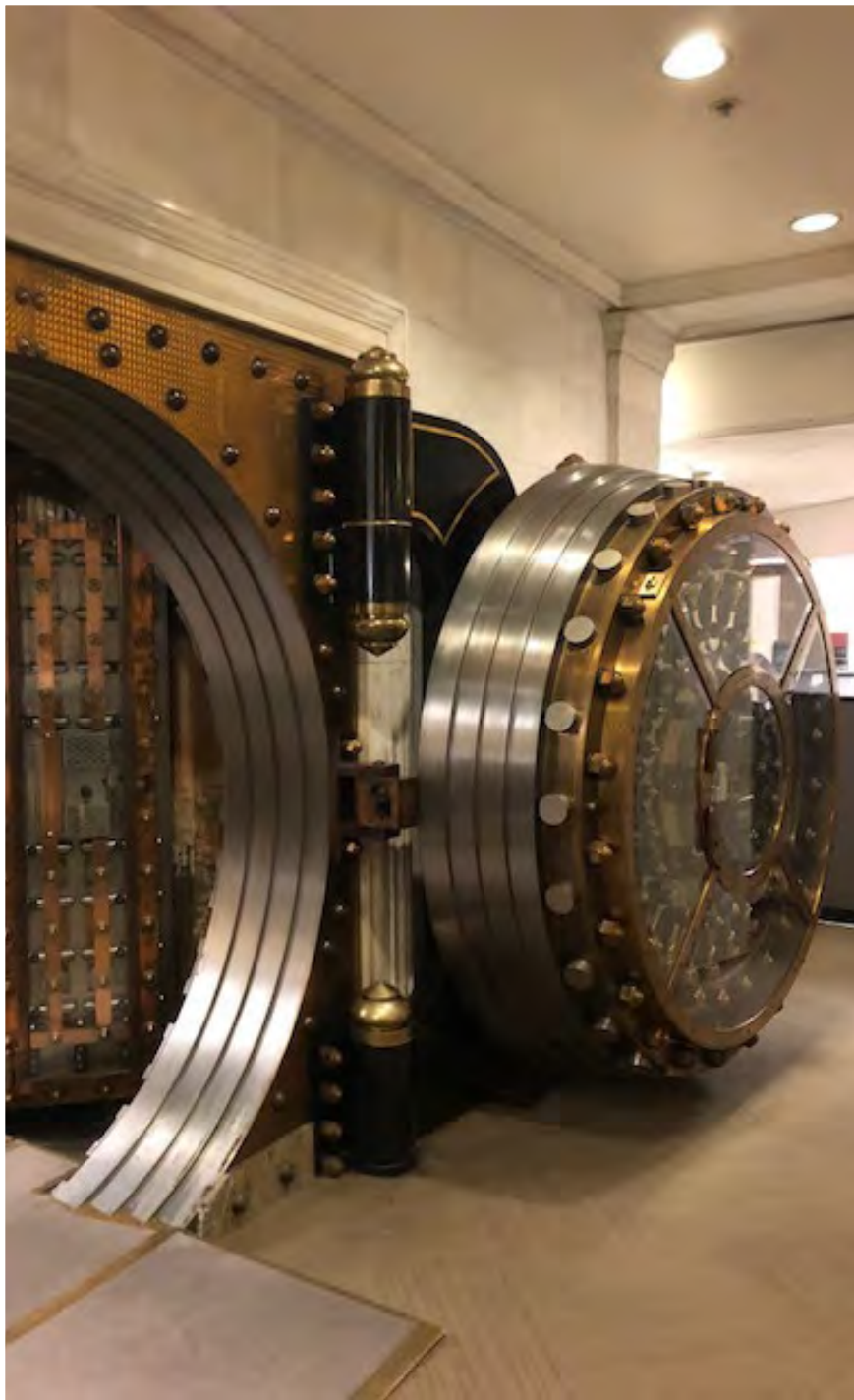
historic vault to remain at basement new floor cuts to provide daylight
