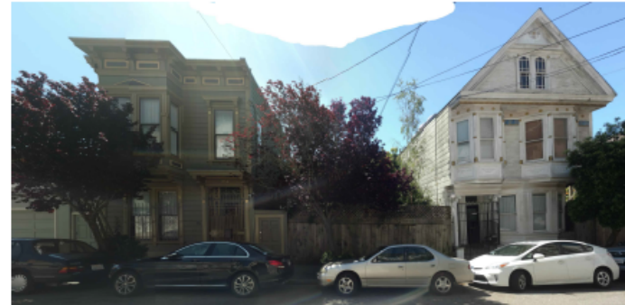
3 SUBJECT PROPERTY & SAME SIDE OF LAUSSAT STREET
