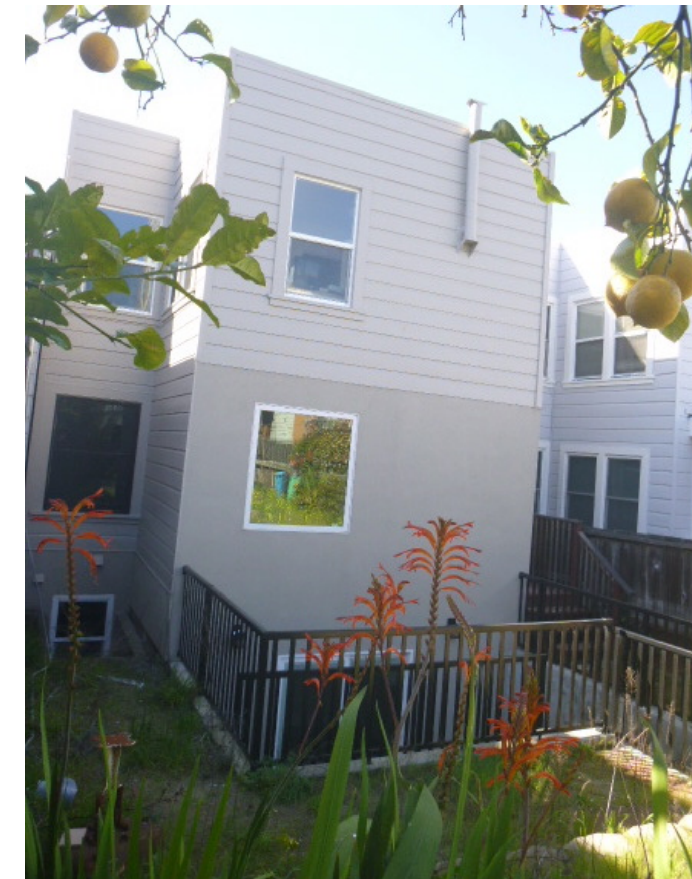
1 REAR VIEW TO NORTH
