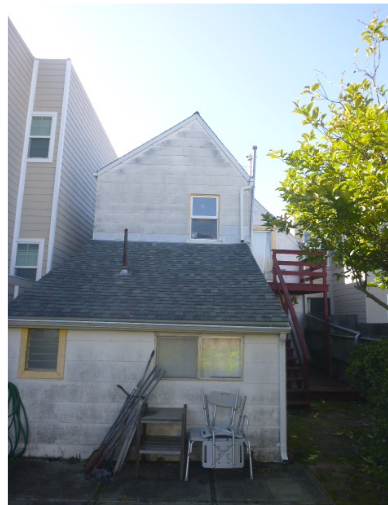
2 EXISTING REAR VIEW
