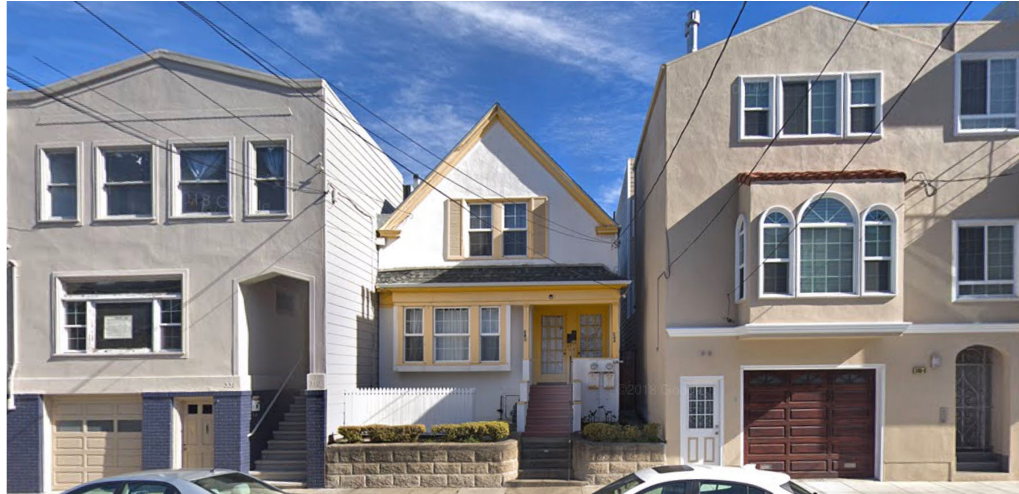
4 EXISTING FRONT VIEW
