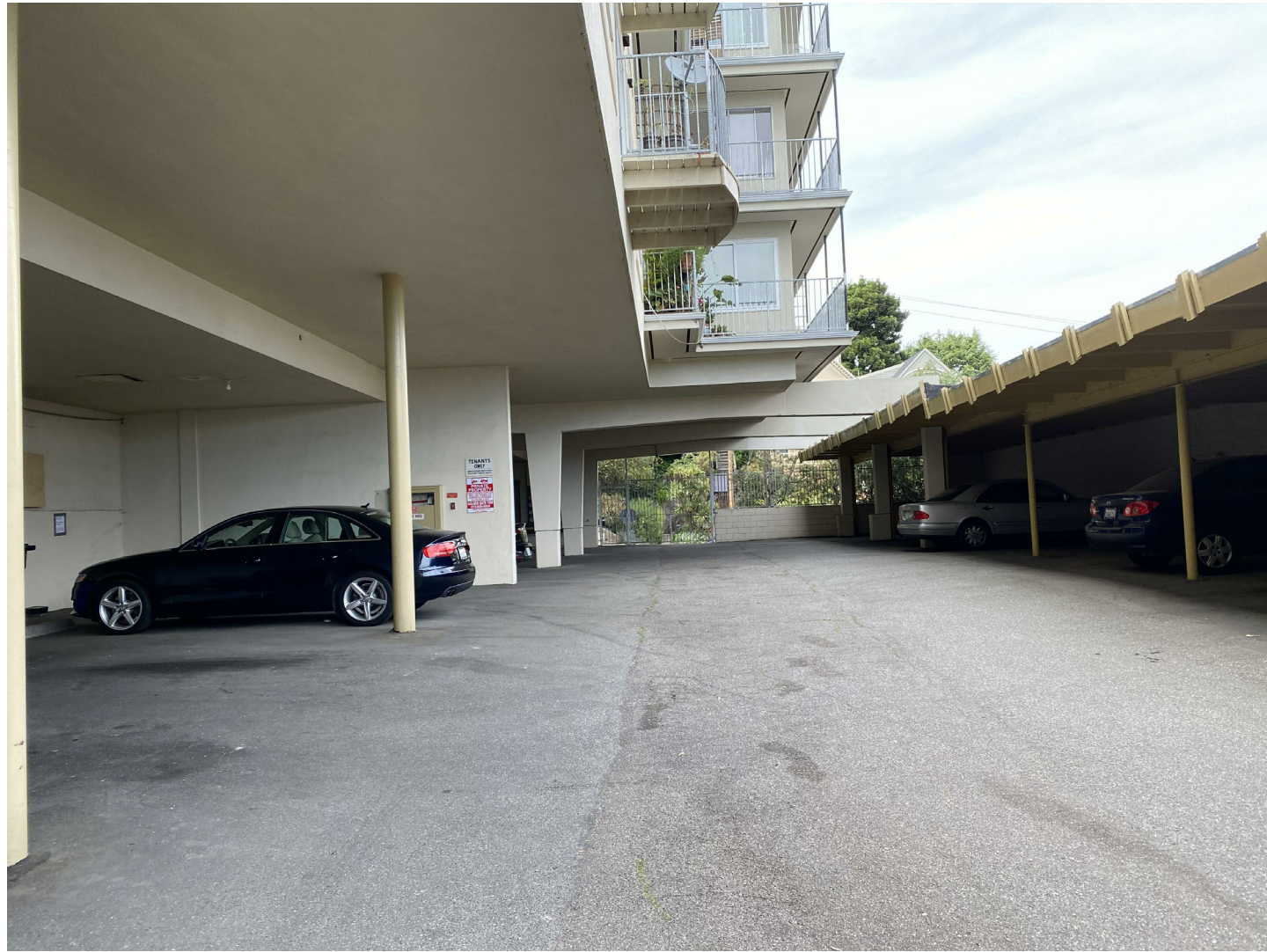
DRIVEWAY LOOKING NORTH
