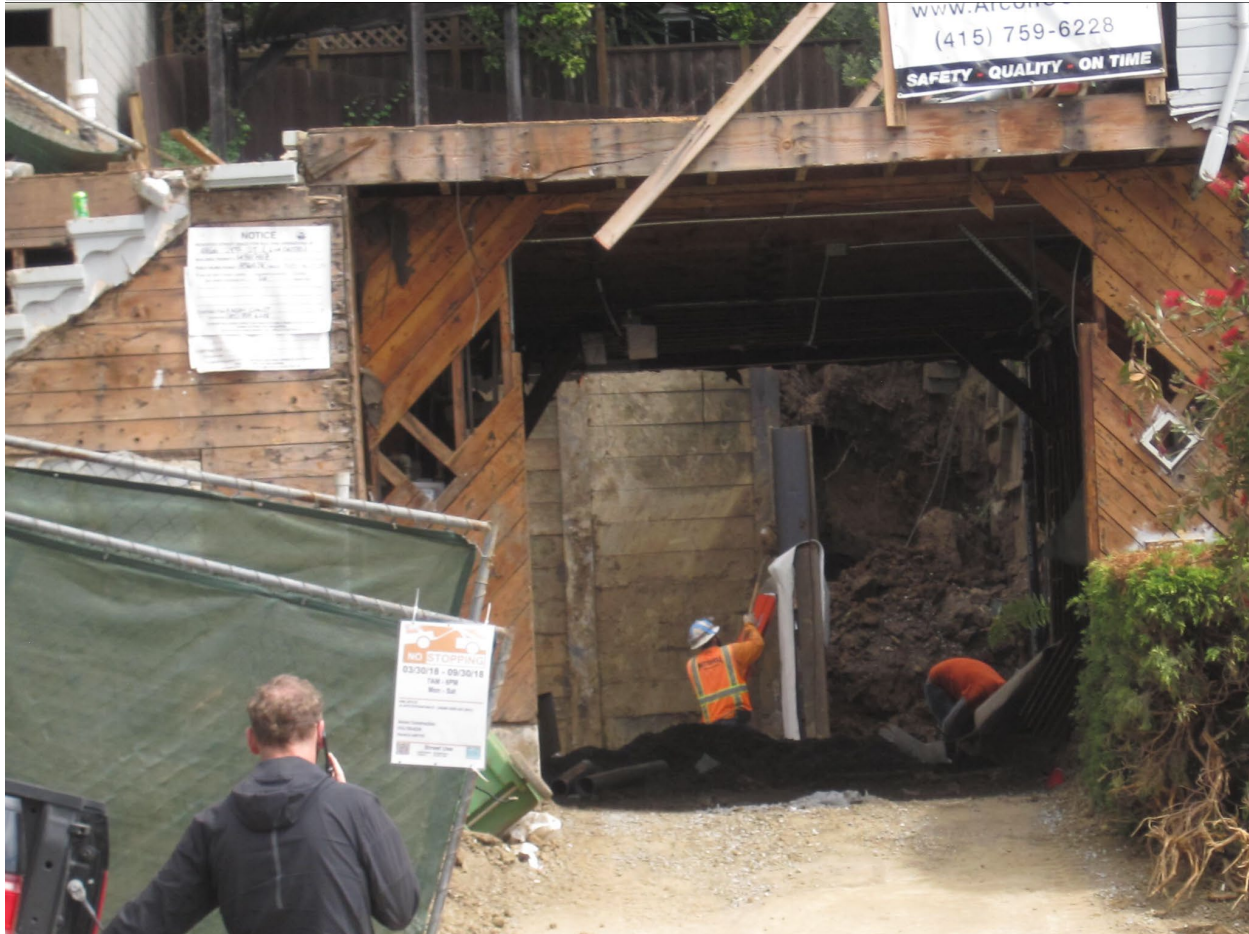
COMPLETED REAR YARD
