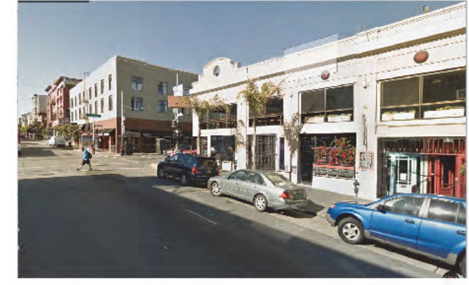
POLK ST. LOOKING NORTHEAST
