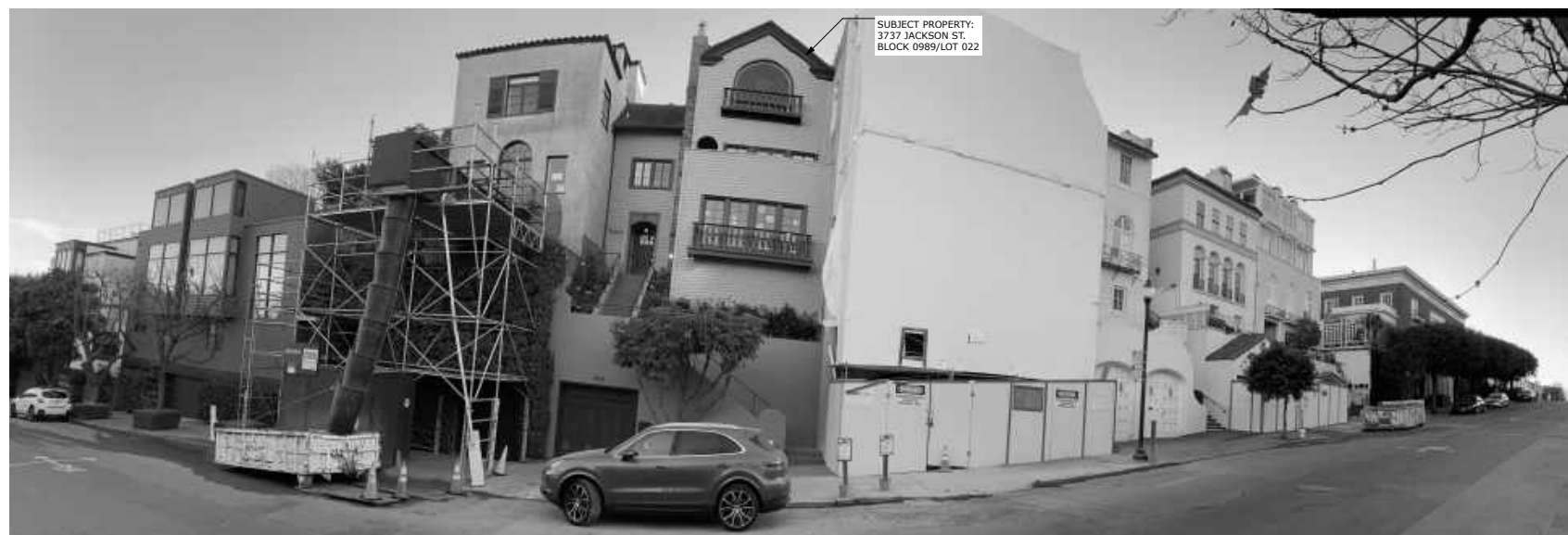
2 PANORAMA VIEW LOOKING SOUTH
