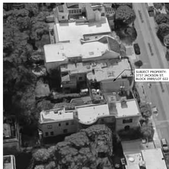
4 AERIAL VIEW LOOKING WEST
