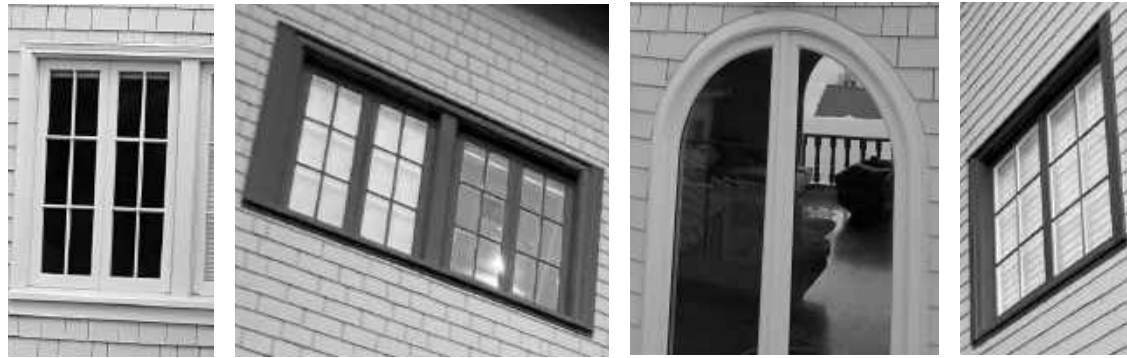
PHOTOS OF (E) WINDOWS
