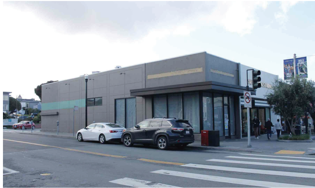
VIEW E: EXISTING FRONT VIEW
