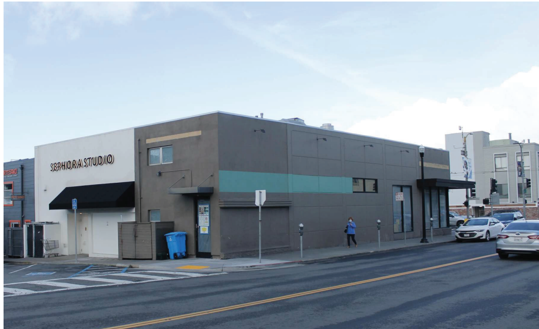
VIEW D: EXISTING REAR VIEW
