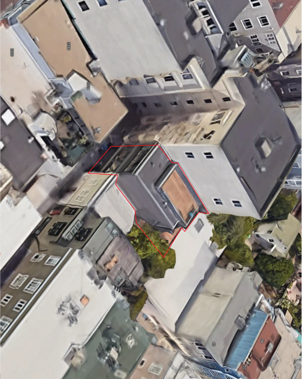
22 Moore Place - Aerial View
