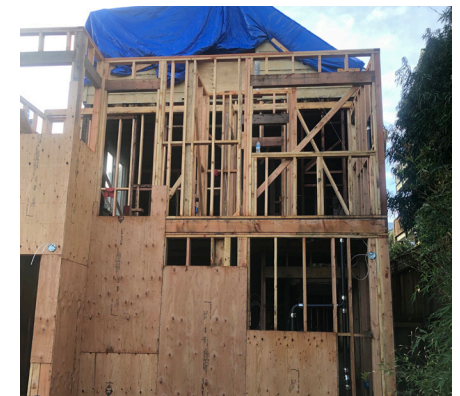
January, 2020 Reframing of upper structure complete and framing inspection signed off.
