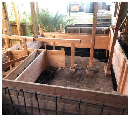
October, 2019 Foundation forms complete for ground floor infill.
