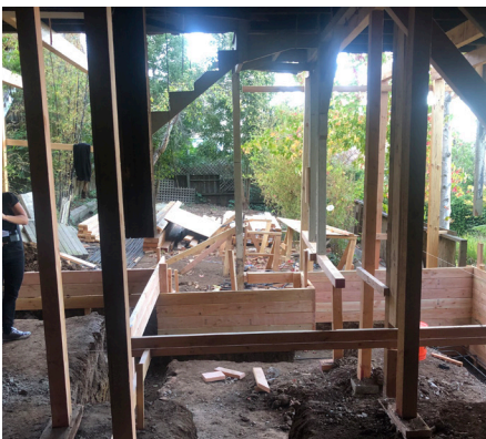
October, 2019 Foundation work being done underneath upper rear structure.
