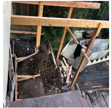
October, 2019 Detail showing support beams holding upper structure in place during infill work.
