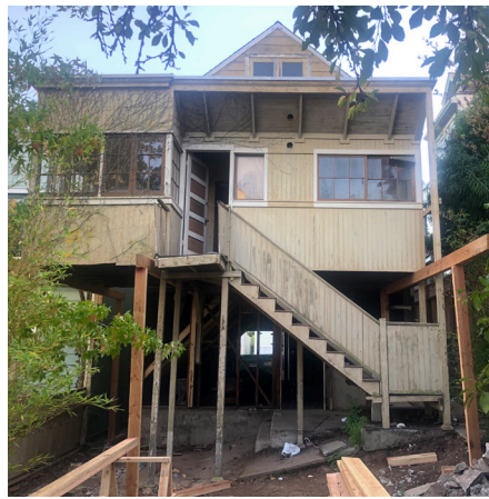
September, 2019 Rear structure supports while infill work underneath began.
