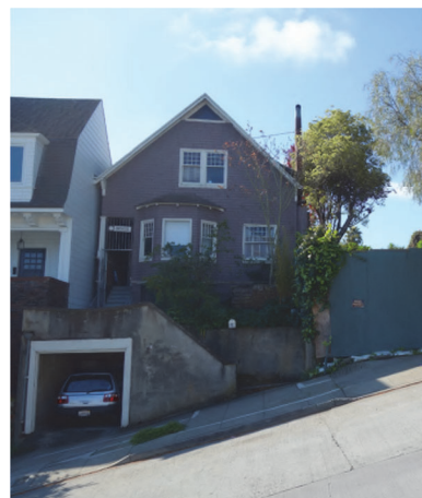
4 FRONT OF ADJACENT BLDG (3663 21ST STREET) N.T.S
