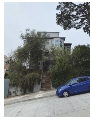
2 FRONT OF ADJACENT BLDG (3677/ 79/ 81 21ST STREET) N.T.S
