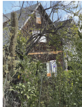
7 REAR OF ADJACENT BLDG (3663 21ST STREET) N.T.S
