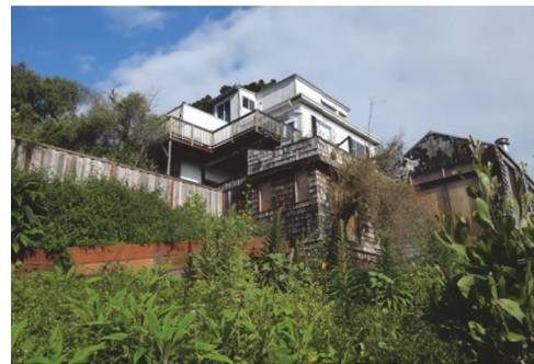
5 REAR OF ADJACENT BLDG (3677/ 79/ 81 21ST STREET) N.T.S
