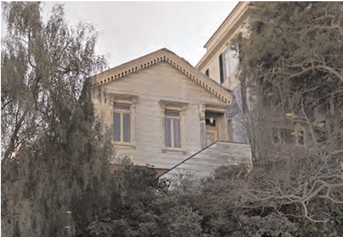
Exhibit 2b below: 3669 21st Street facade in recent photograph.
