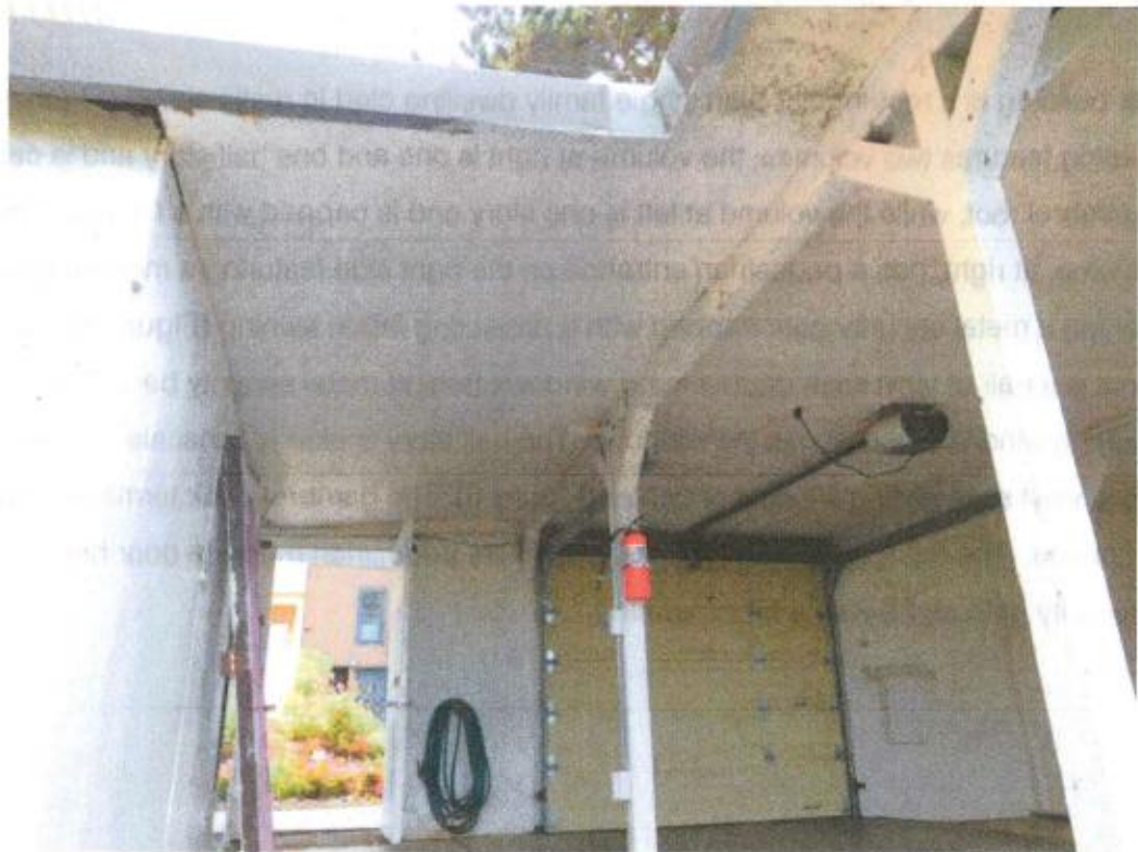
Figure 2: 617 Sanchez Street, front carport, interior
