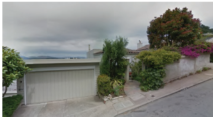
6 FRONT OF OPPOSITE BLDG'S (40 & 50 BELGRAVE) N.T.S
