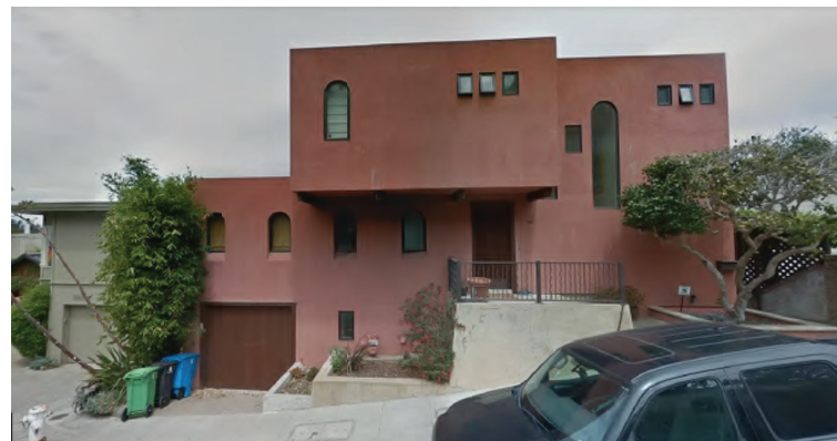
8 FRONT OF OPPOSITE BLDG'S (60 BELGRAVE) N.T.S
