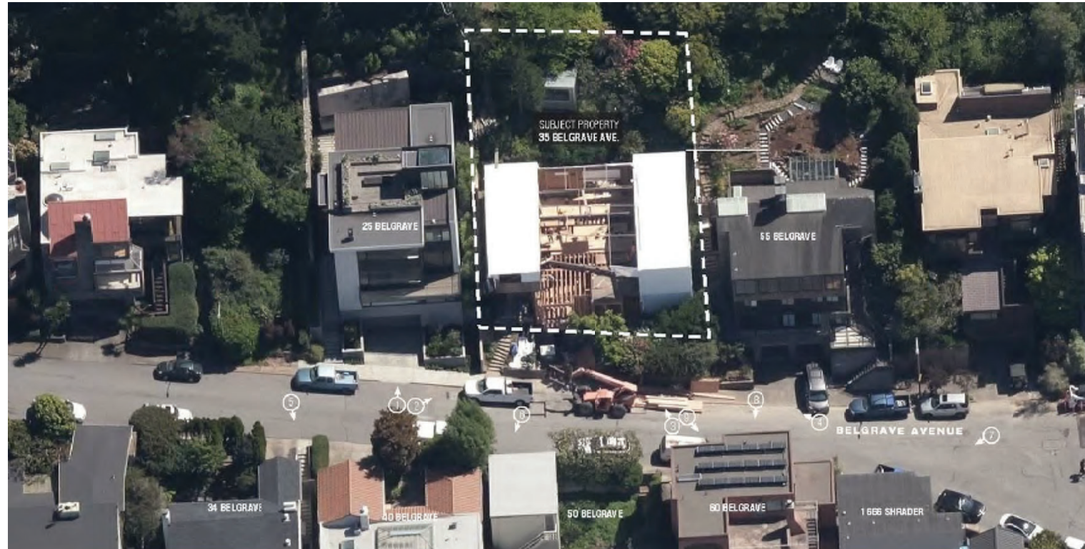
10 AERIAL PHOTOGRAPH N.T.S
