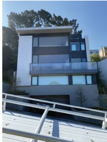
1 FRONT OF ADJACENT BLDG (25 BELGRAVE) N.T.S
