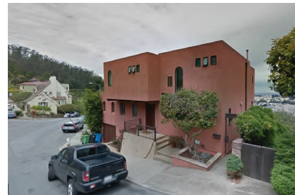
9 FRONT OF OPPOSITE BLDG'S (60 BELGRAVE) N.T.S
