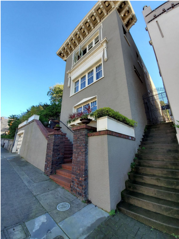
Primary and west facade, looking southeast.
