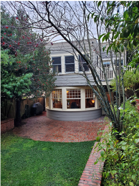
Rear facade, looking northwest.
