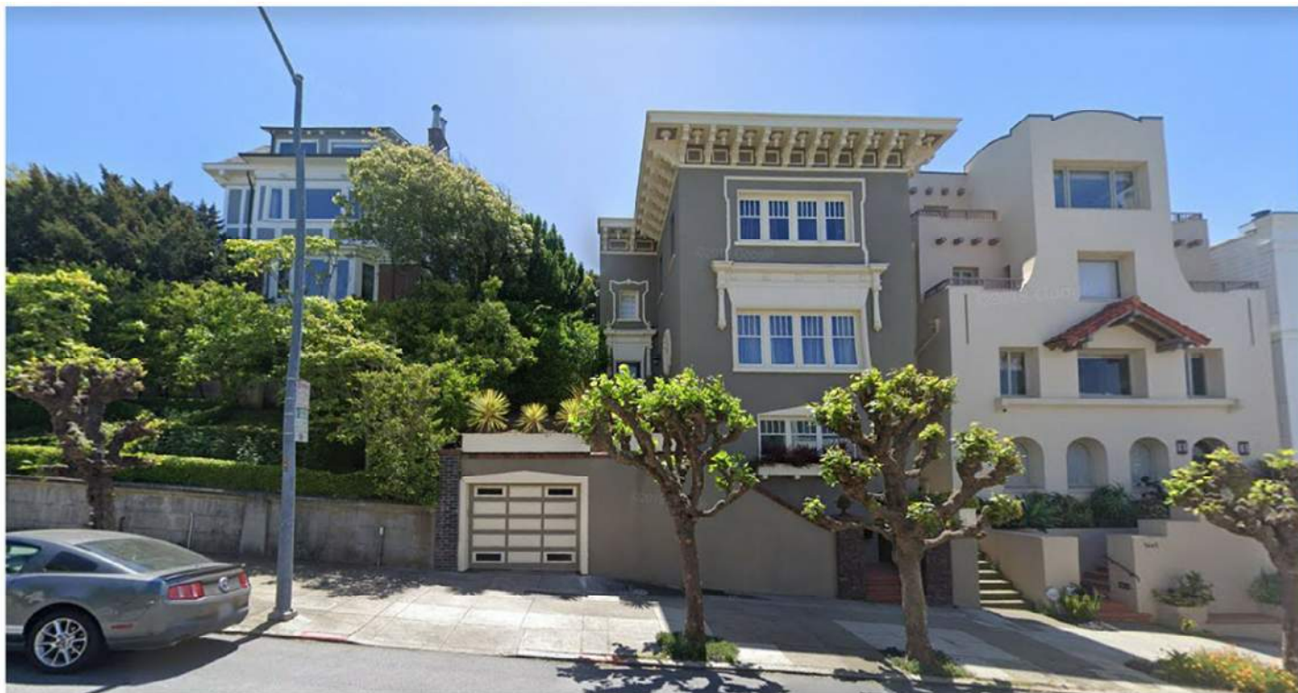
MASSING VIEW 01 - EXISTING VIEW FROM FRONT OF HOUSE
