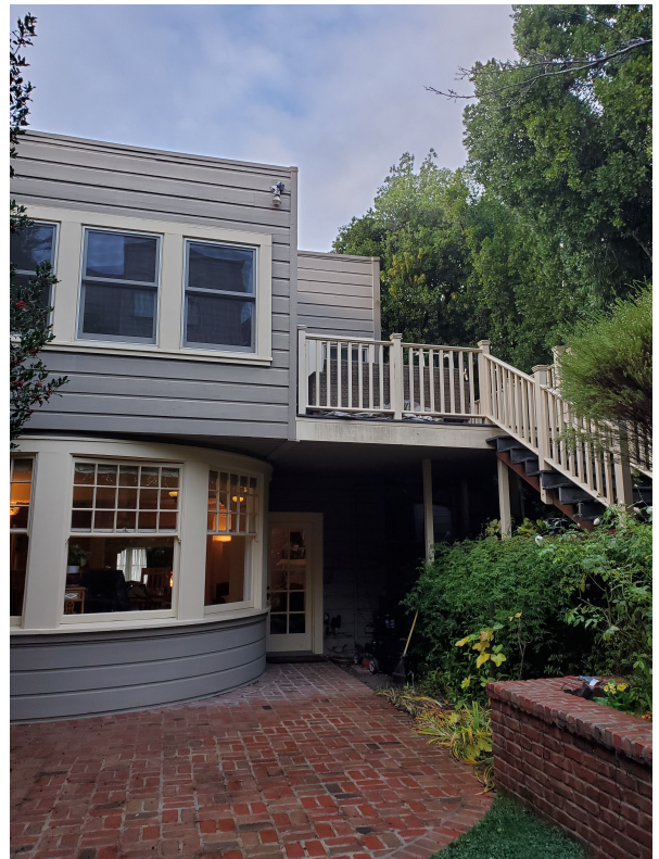
Right side of rear facade, looking northeast.
