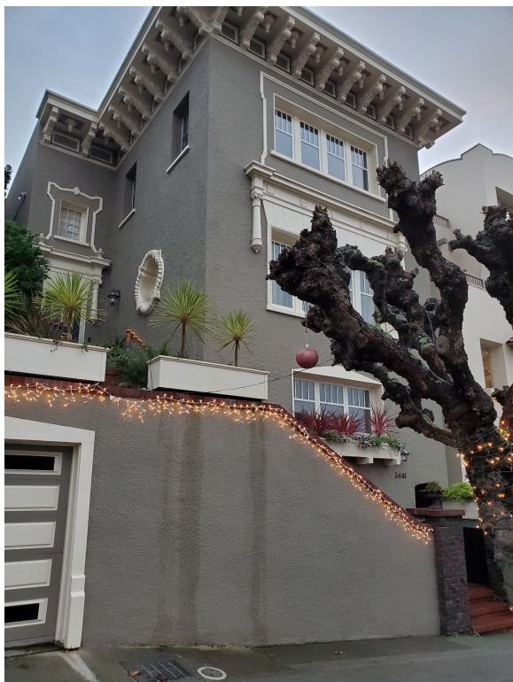
Right side of primary facade, looking southwest.
