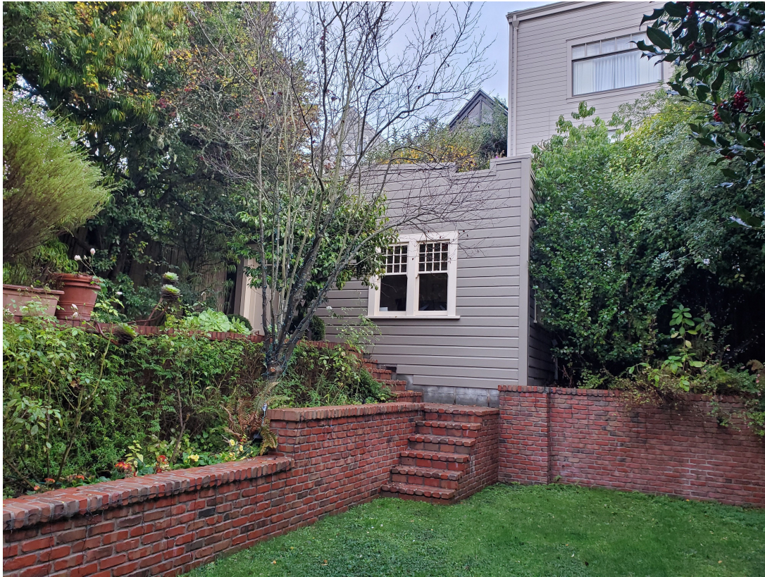
Auxiliary building, looking southeast from backyard.
