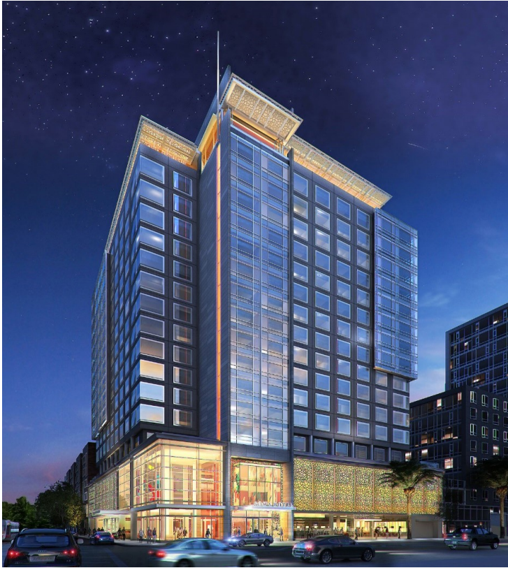
SOMA Hotel Project 100 Channel Street Mission Bay Block 1
