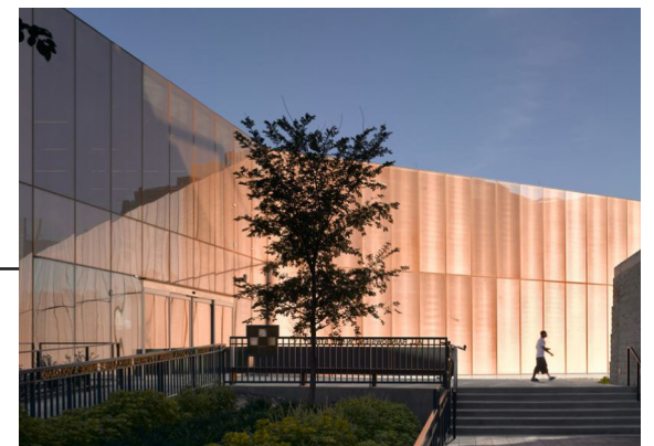
UNITIZED CURTAIN WALL W/ EXPANDED METAL SANDWICHED GLAZING (DARK BRONZE ANODIZED ALUMINUM)
