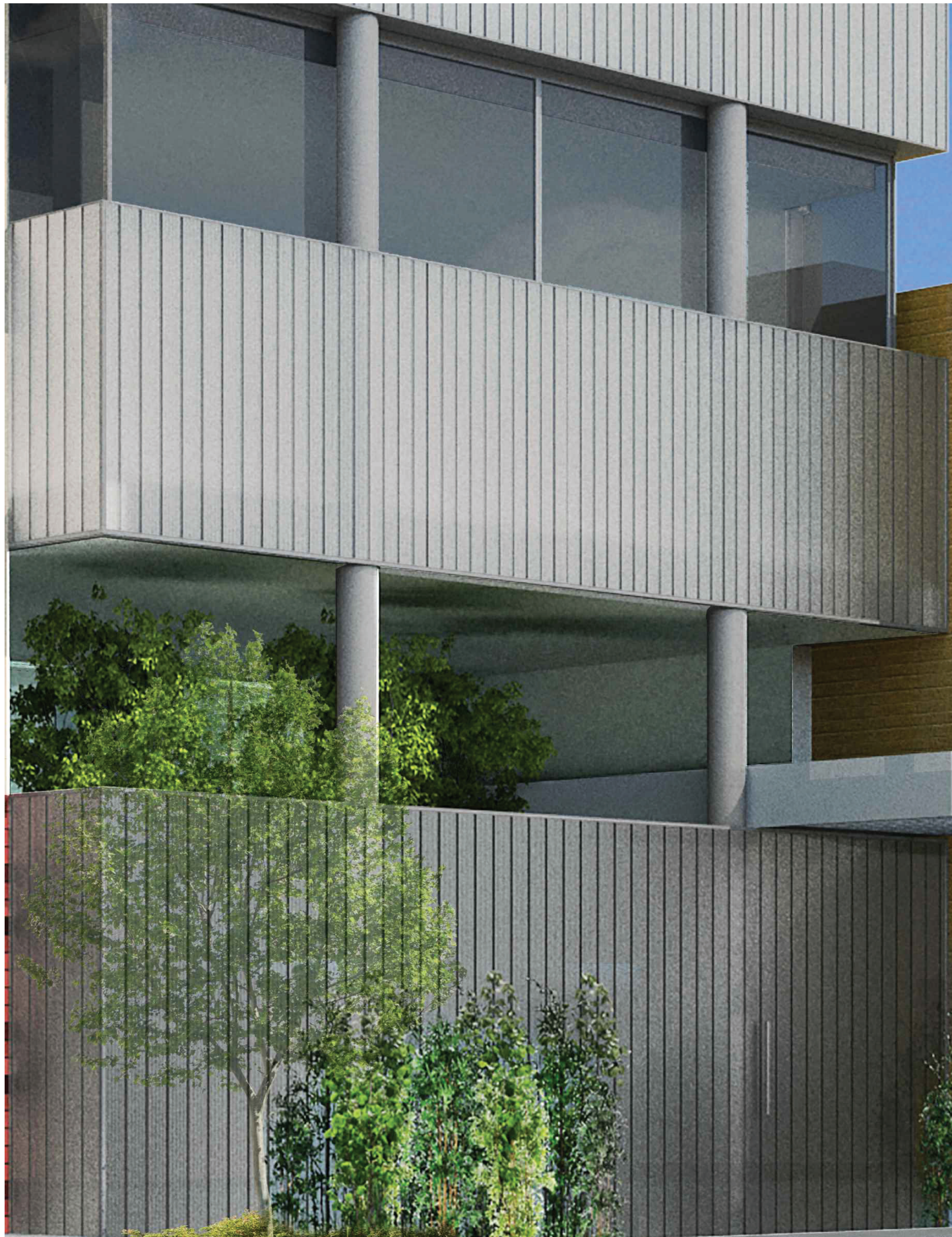
LINEAR SIDING DETAIL VIEW 1
