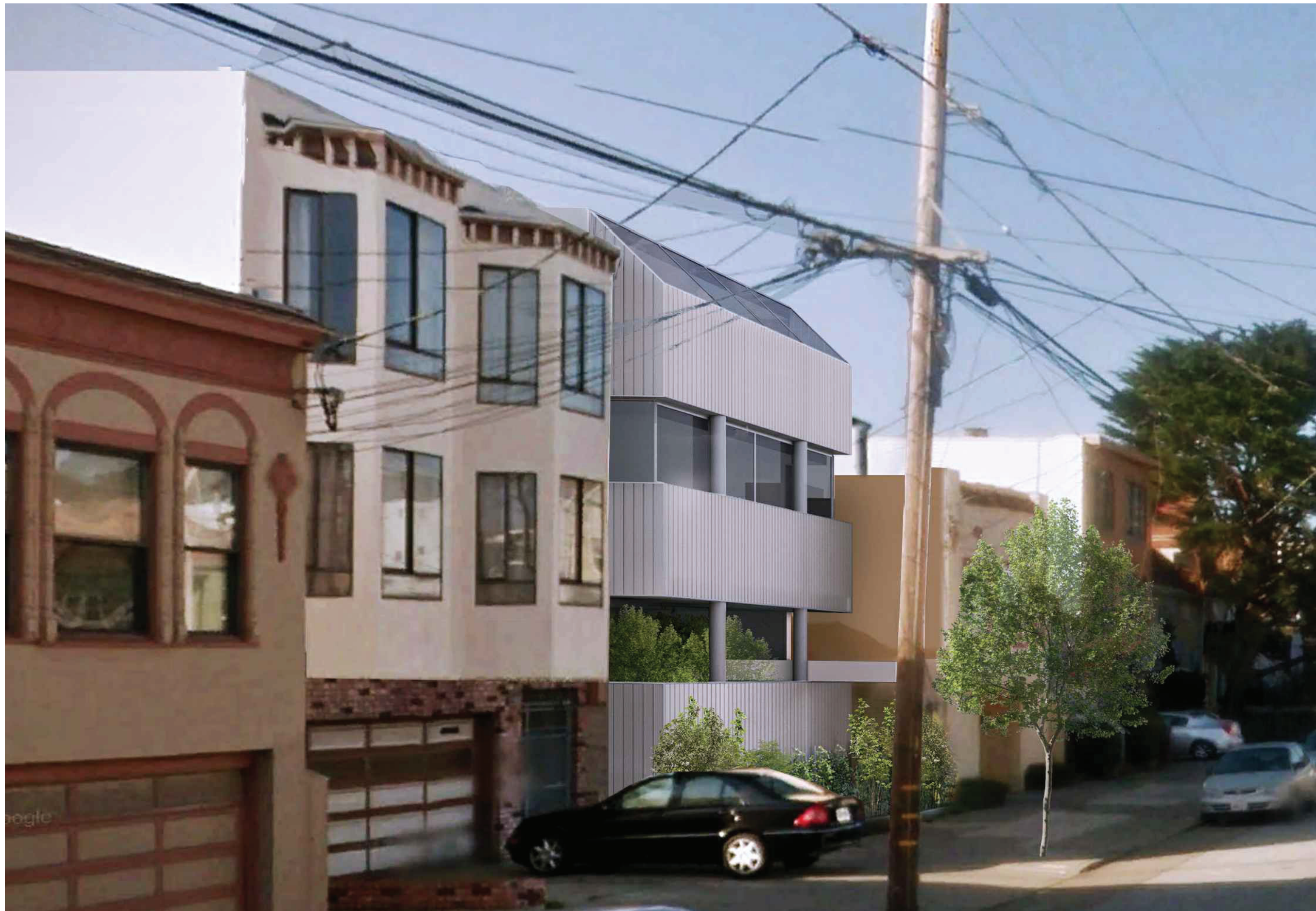
VIEW FROM 46TH STREET 1
