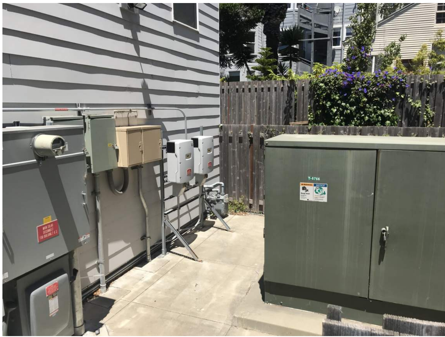
Photo of PG&E Transformer, Electrical Panel, and Solar Inverters
