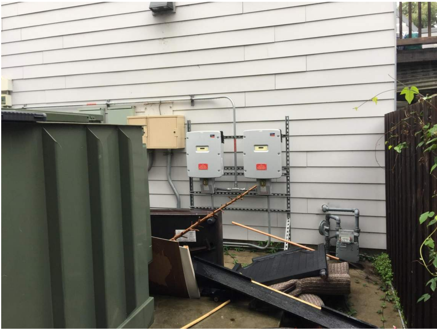
Photo of More Solar Inverters and Gas Utility Location
