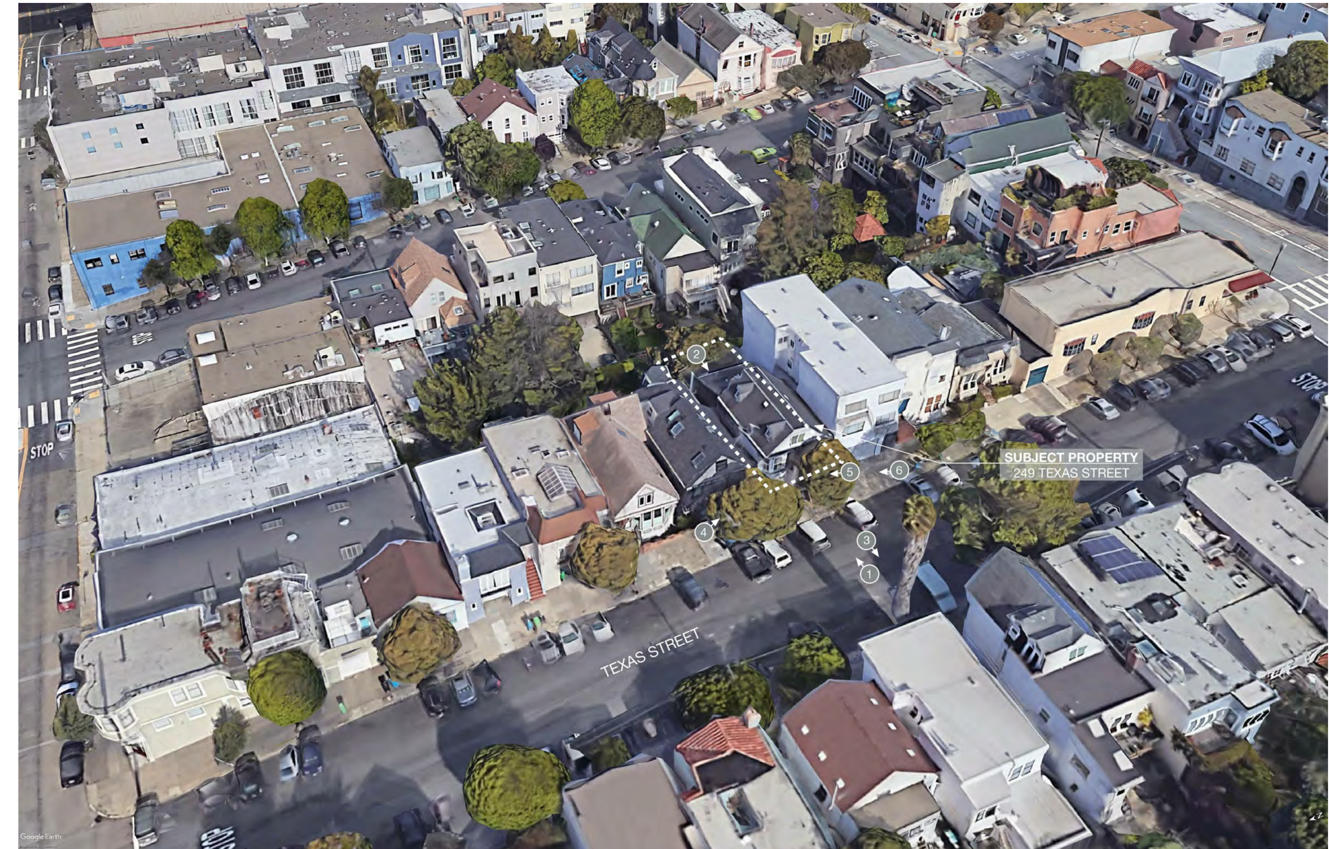
0 AERIAL - PHOTO LOCATION KEY
