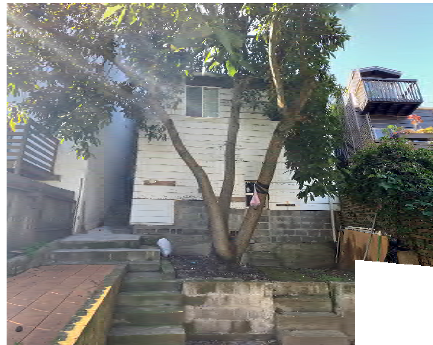
2 REAR FACADE OF SUB. PROP. & NEIGHBORS
