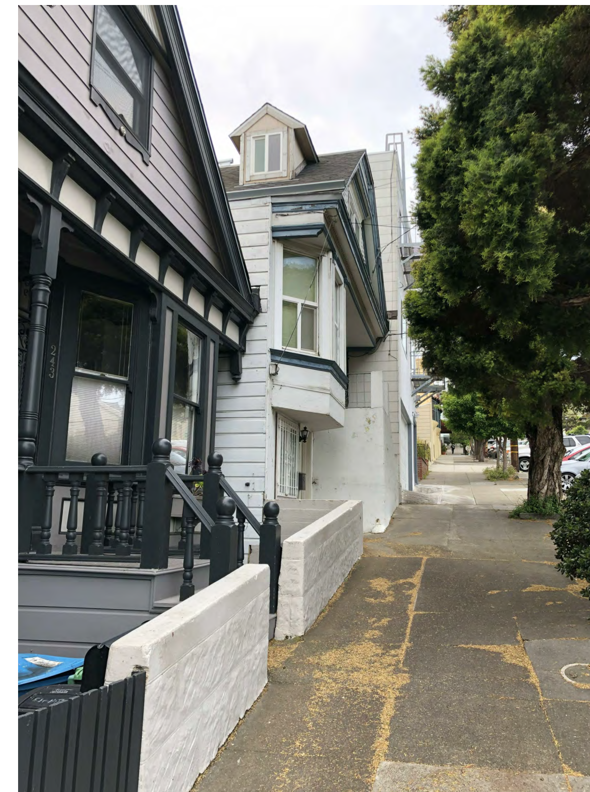
4 SIDE FACADE OF SUBJECT PROPERTY
