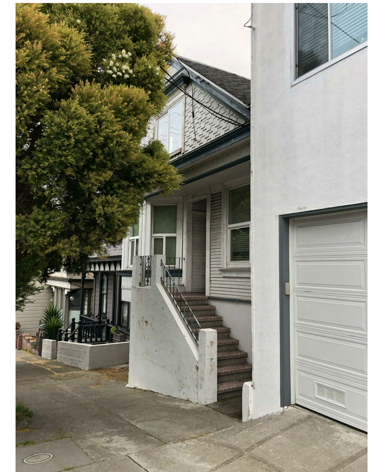
5 SIDE FACADE OF SUBJECT PROPERTY
