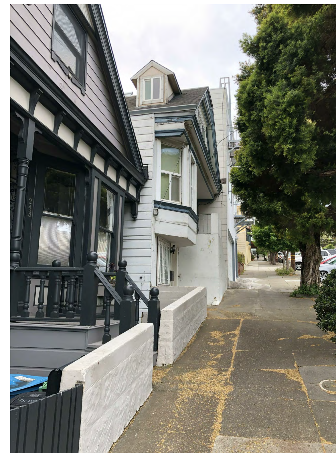
4 SIDE FACADE OF SUBJECT PROPERTY
