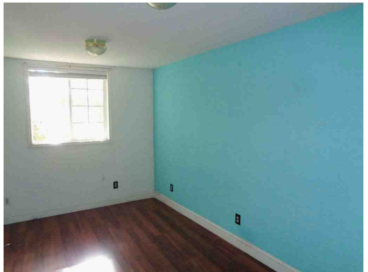
Lower Level Rooms
