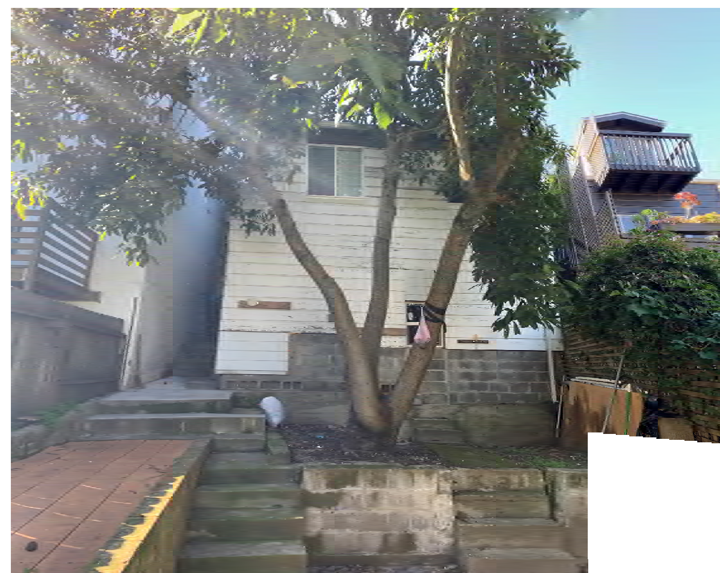
2 REAR FACADE OF SUB. PROP. & NEIGHBORS
