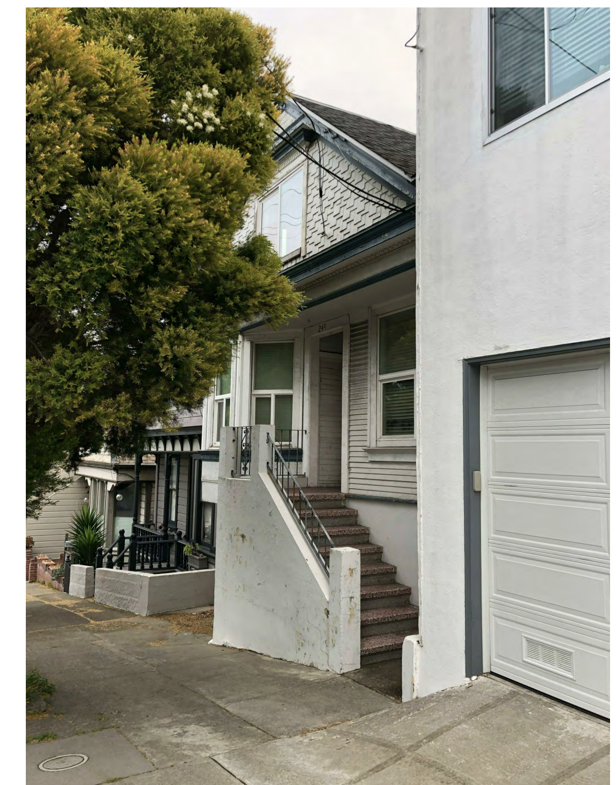
5 SIDE FACADE OF SUBJECT PROPERTY
