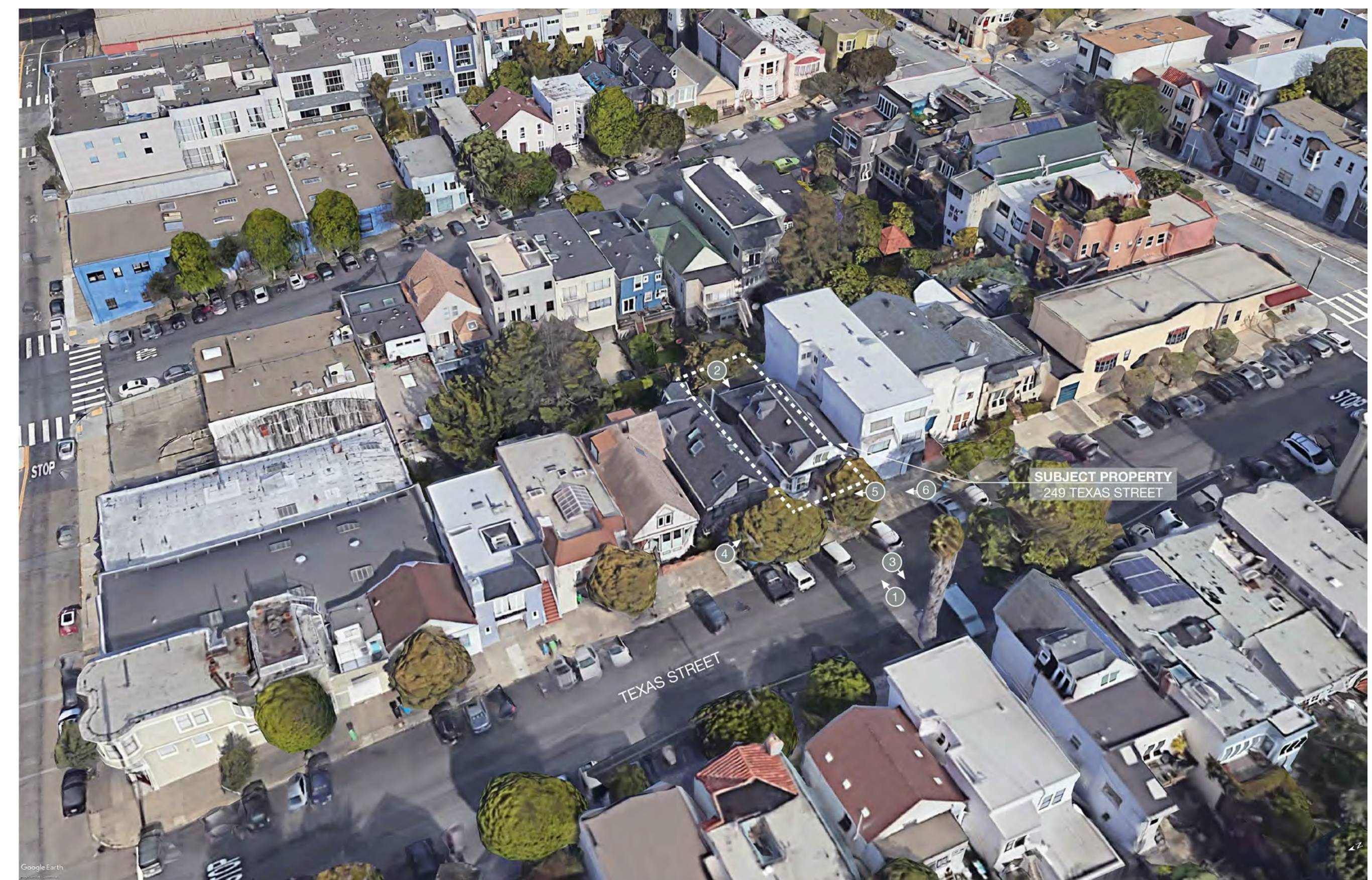
0 AERIAL - PHOTO LOCATION KEY
