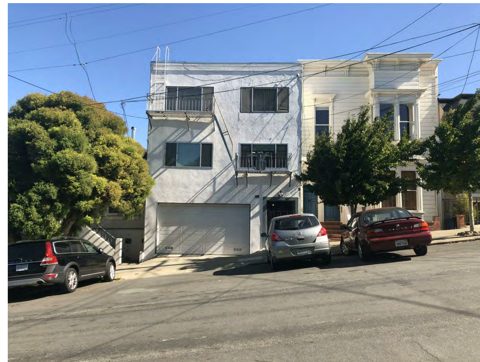
1b FRONT FACADE OF ADJ. BLDG, 243 TEXAS
