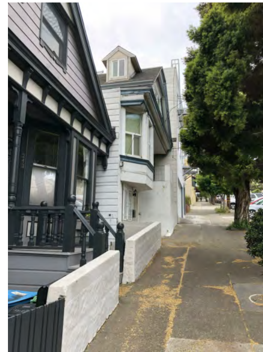
4 SIDE FACADE OF SUBJECT PROPERTY 1/4" = 1'-0"
