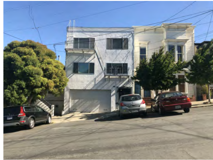
1b FRONT FACADE OF ADJ. BLDG, 243 TEXAS 1/4" = 1'-0"
