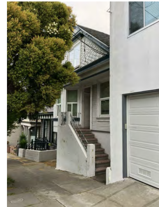
5 SIDE FACADE OF SUBJECT PROPERTY 1/4" = 1'-0"
