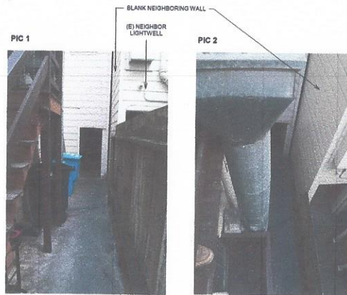
(E) LIGHTWELL @ WEST SIDE
