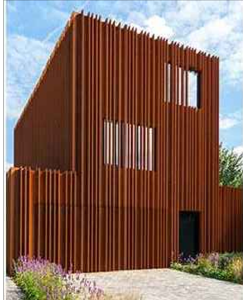
Corten steel sections for areas of exterior fenestration Matte Finish
