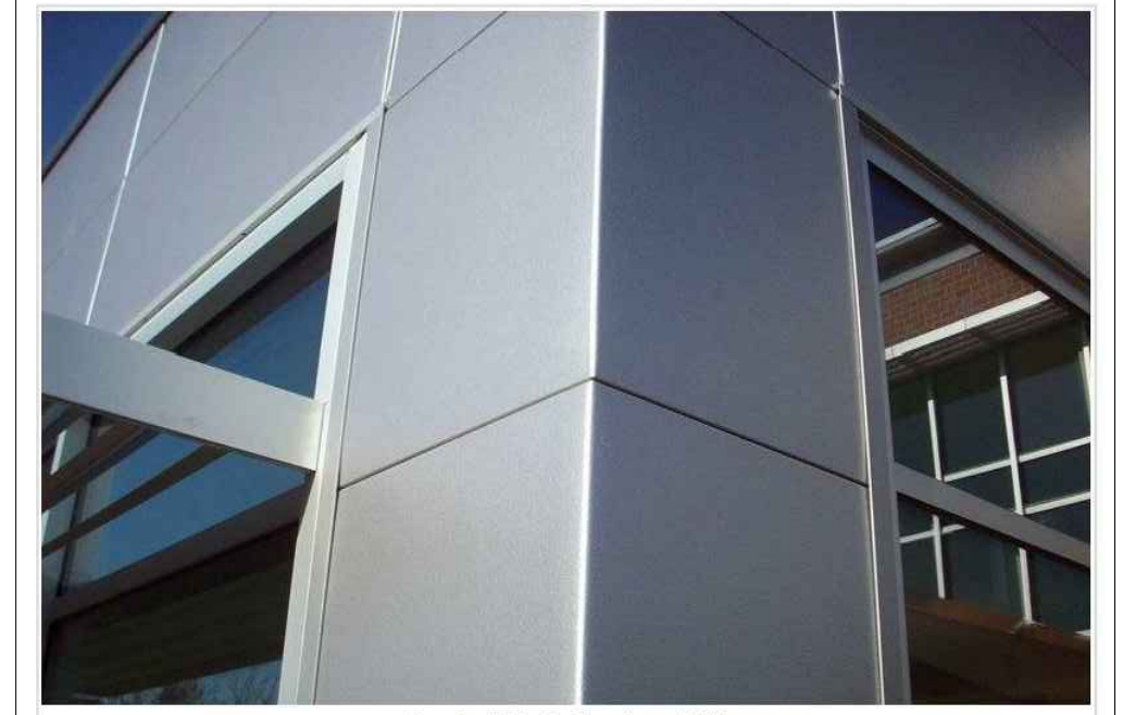
Matte finished Anodized Aluminum panel system & non-reflective glazing
