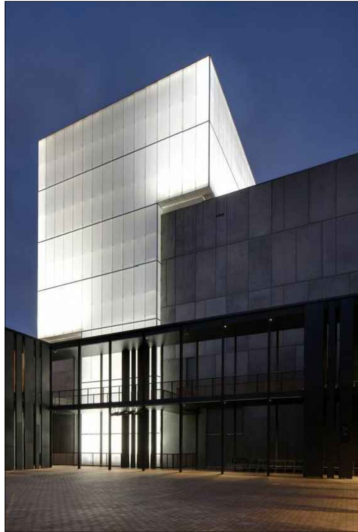
Non-reflective Cast Glass rear stair enclosure with Matte finished Anodized Aluminum frames
