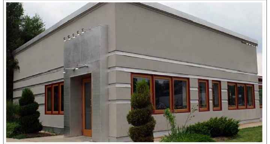
Smooth cement stucco & metal shadow gap jointing to exterior Matte Finish
