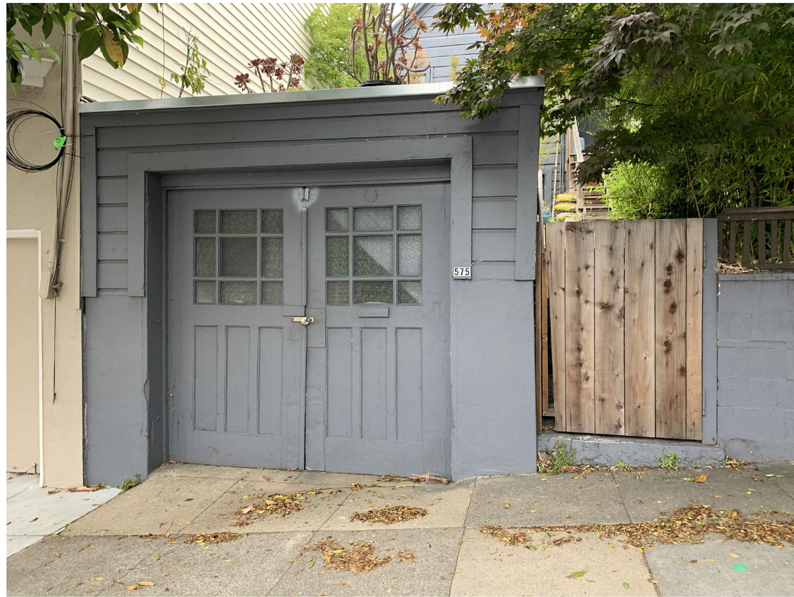
PHOTO 'A' - FRONT VIEW AT STREET: SUBJECT PROPERTY DETACHED GARAGE
