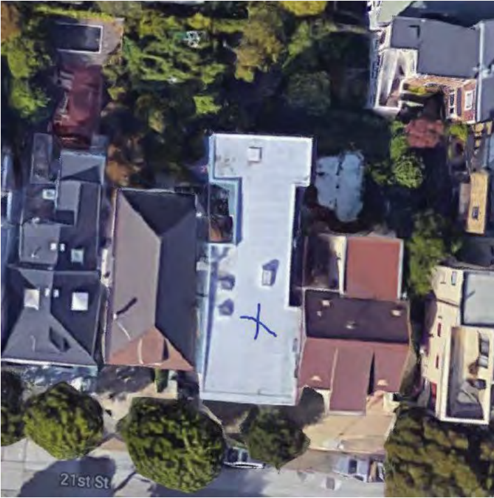
Aerial prior to alterations
