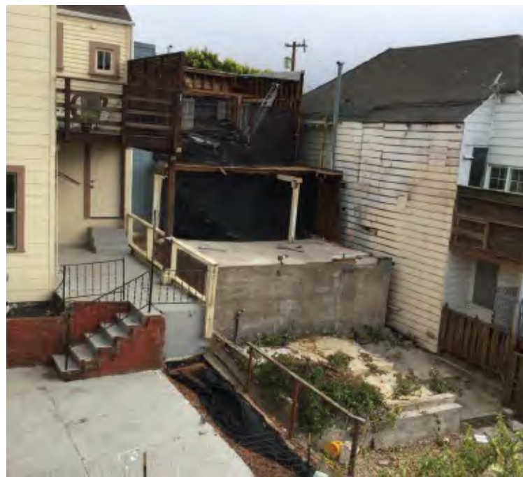
Rear of subject building during alterations
