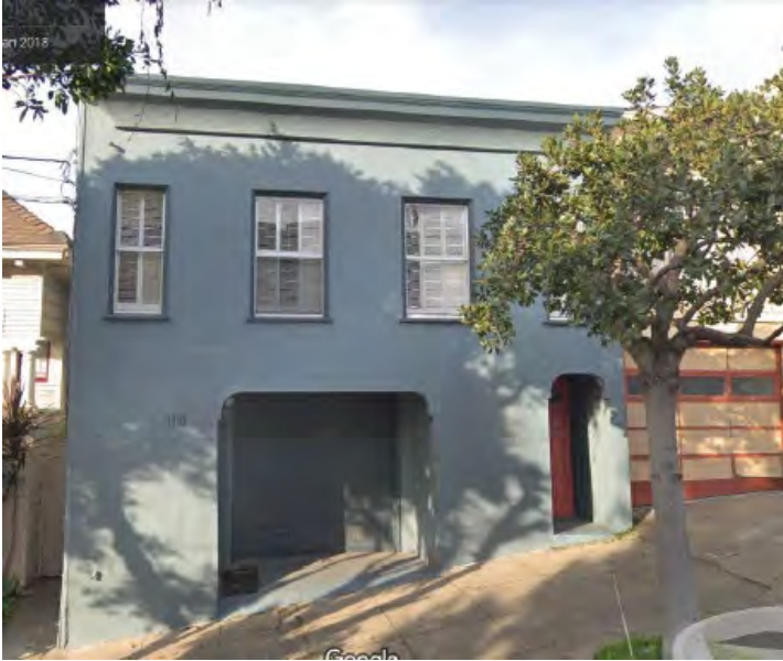
Front of subject building prior to alterations
