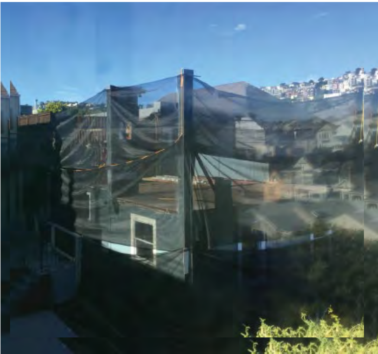
Rear of subject building during alterations
