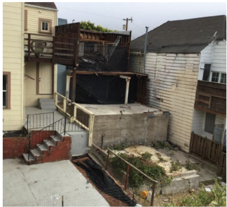
Rear of subject building during alterations
