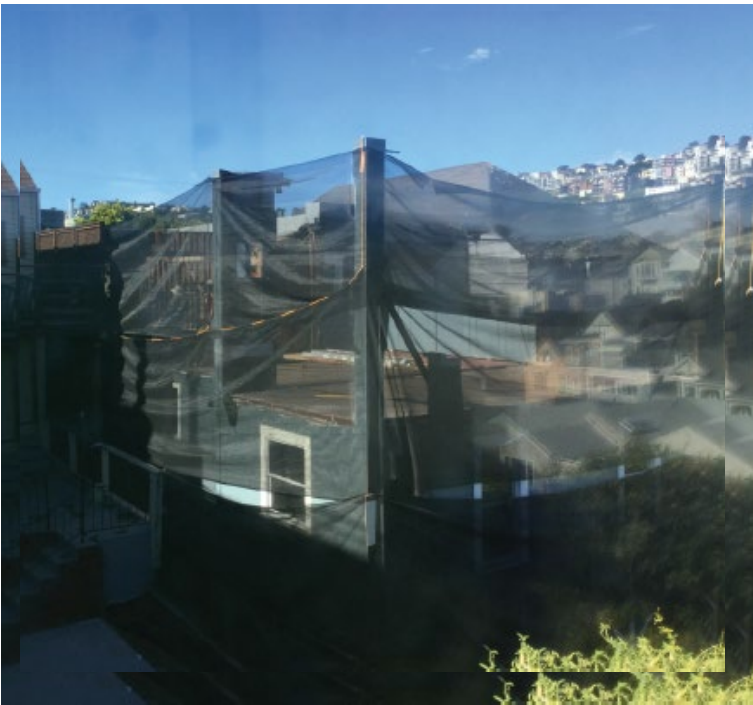
Rear of subject building during alterations
