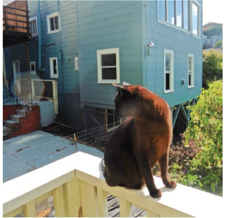
Rear of subject building prior to alterations
