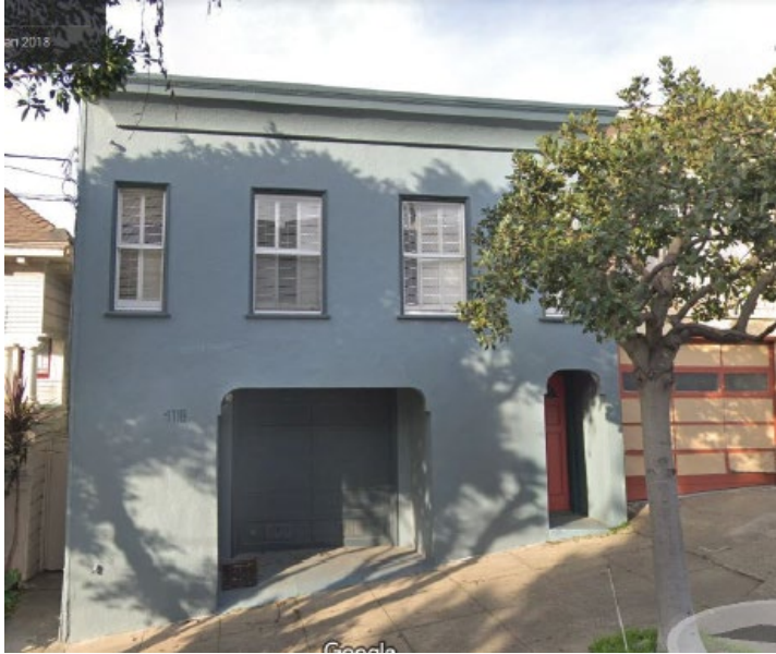
Front of subject building prior to alterations
