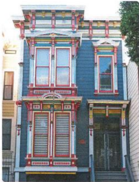
Victorian buildings provide an opportunity for vibrant facade expressions.
