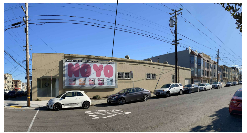
2 BUILDINGS ON THE SAME SIDE OF THE STREET ( 32ND AVENUE )
