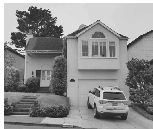
SUBJECT PROPERTY 24 ROSEWOOD DRIVE
