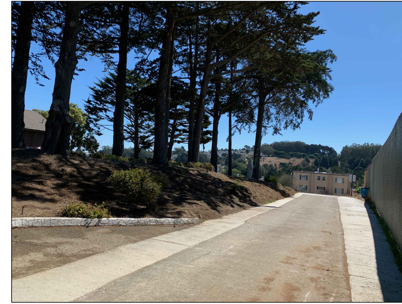
THE SITE FACING THE BACON ST
