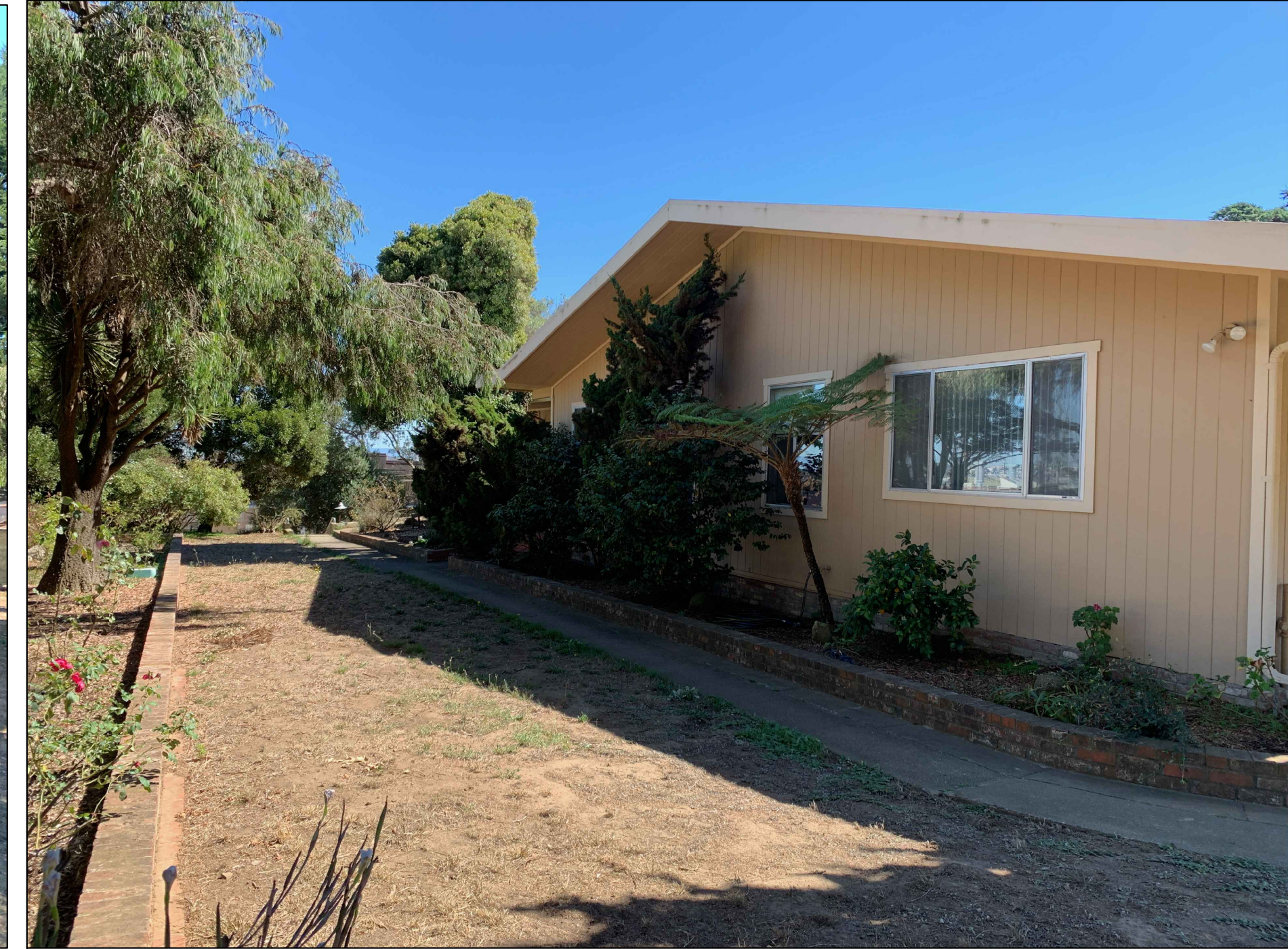
EXISTING BUILDING FRONT ELEVATION 2
