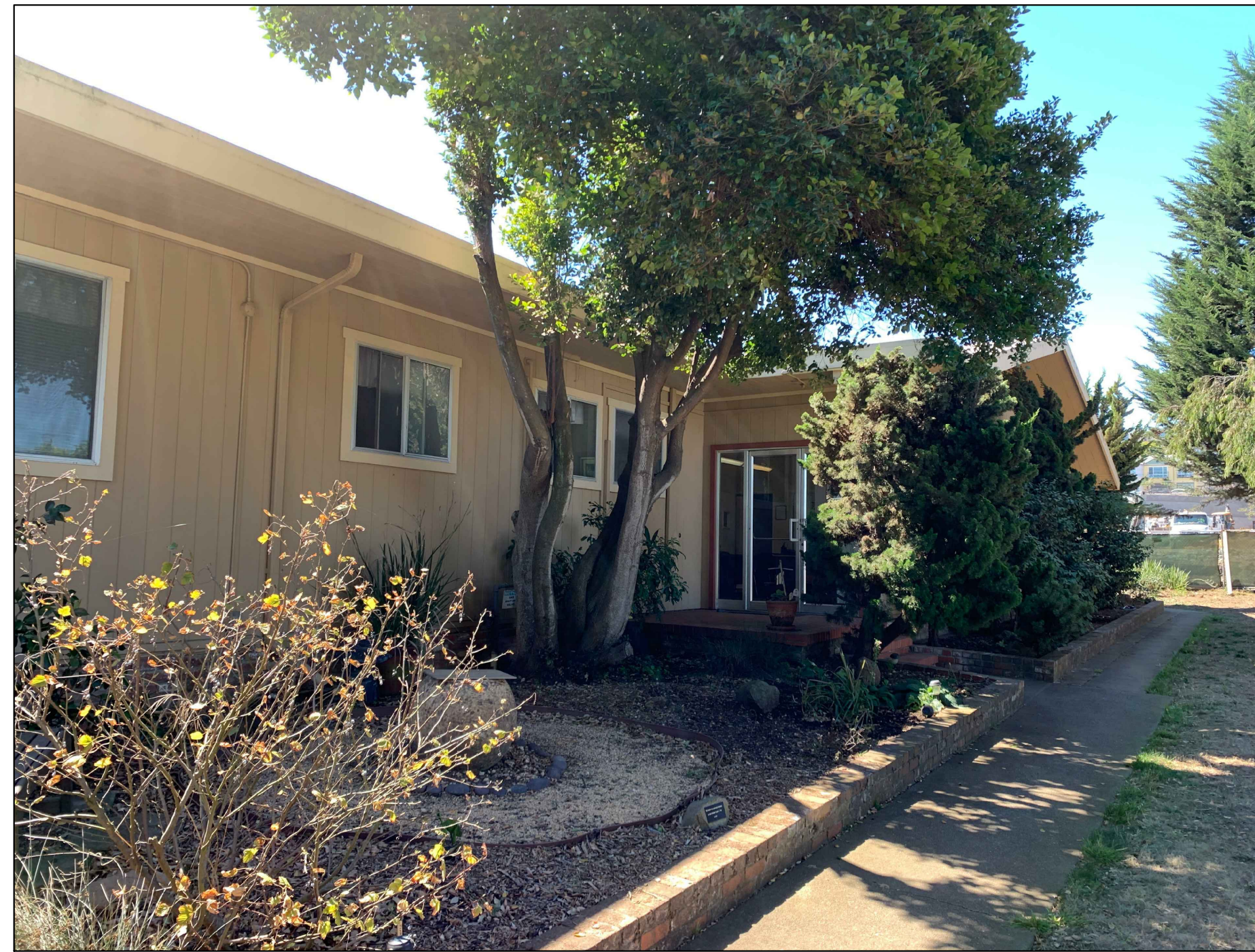
EXISTING BUILDING FRONT ELEVATION 1
