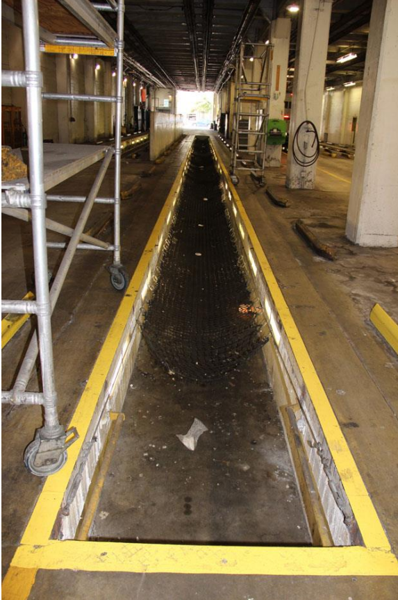
Figure 55. Maintenance pit, looking south.
