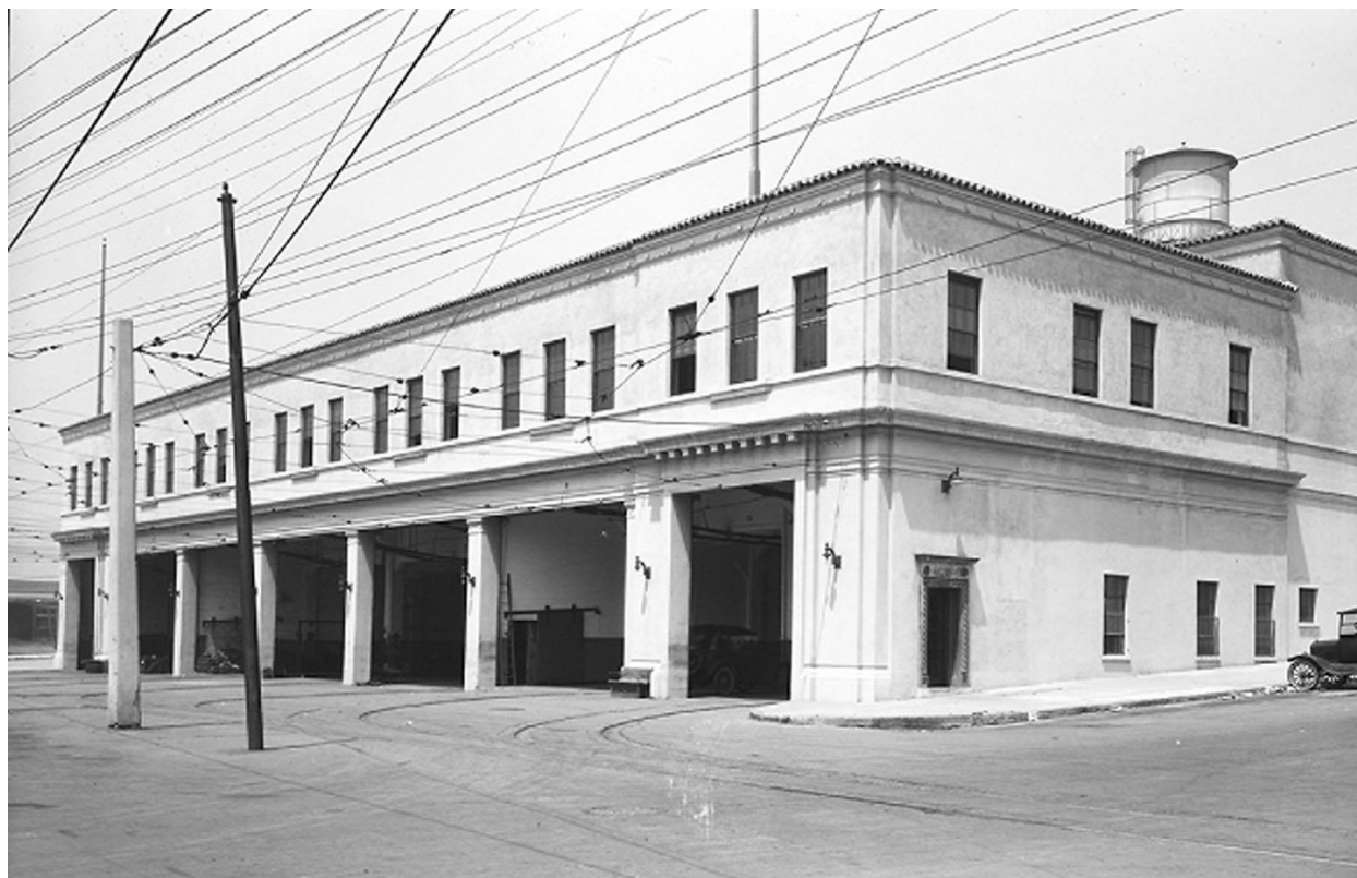
Figure 77. Mariposa Street façade of Potrero Car Barn, May 12, 1926. Source: SFMTA Photography Department and Archive, Image No. W10351
