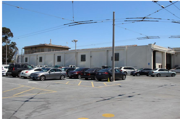
Figure 27. Parking deck, looking northeast.
