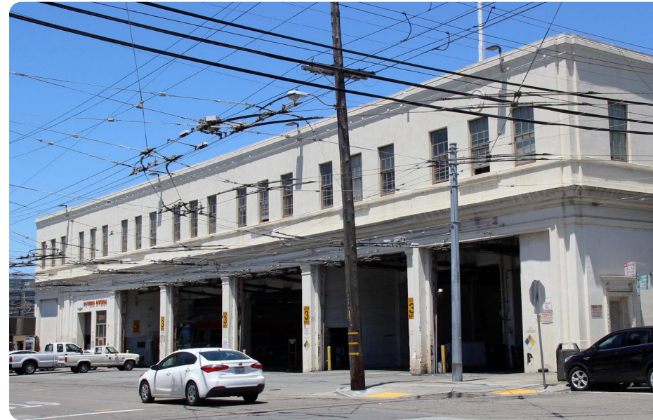
Image 2: View northwest of office wing primary façade along Mariposa Street (left), and secondary façade along Hampshire Street (right).
