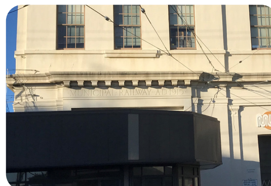
Image 8: Detail view of office wing primary façade. Note character-defining features include remaining door trim of westernmost bay.
