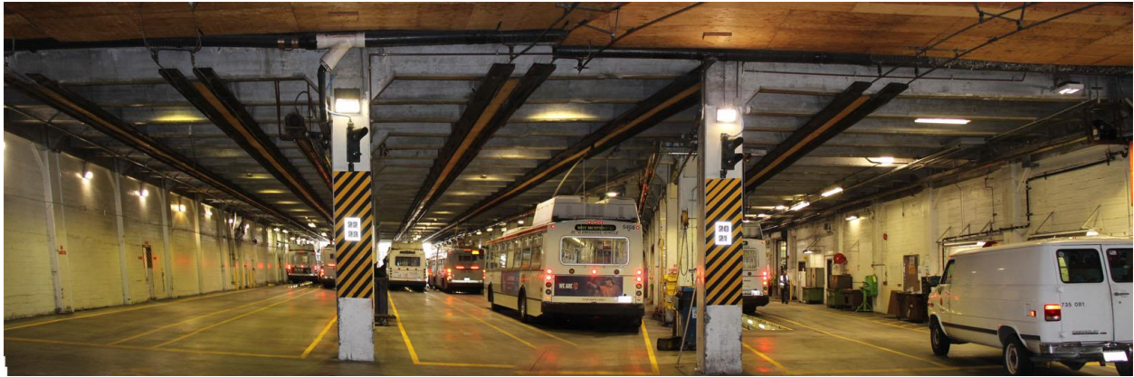
Figure 53. Maintenance bays, looking south.
