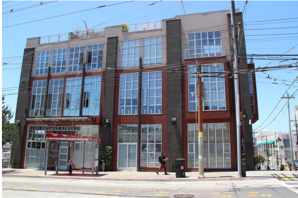
Figure 12. 1800 Bryant Street, looking west.
