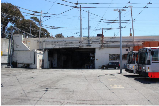
Figure 49. Vehicular entrance at north end of west façade, looking east from bus yard.
