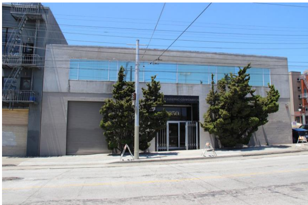
Figure 10. 1850 Bryant Street, looking west.
