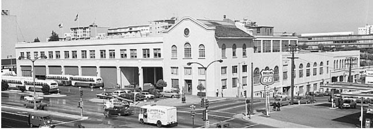
Figure 89. Geary Street Car Barn at Geary Boulevard and Presidio Avenue, 1968; built 1912. Source: SFMTA Photography Department and Archive, Image No. M0324_2
