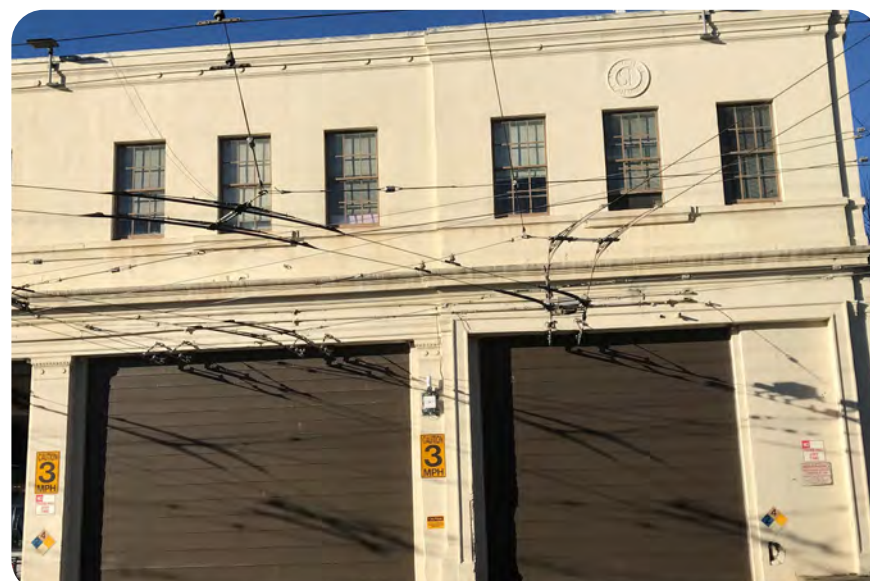
Image 9: Detail view of office wing primary façade. Note character-defining features include large vehicular openings, double-hung windows, and medallion featuring original Muni logo.
