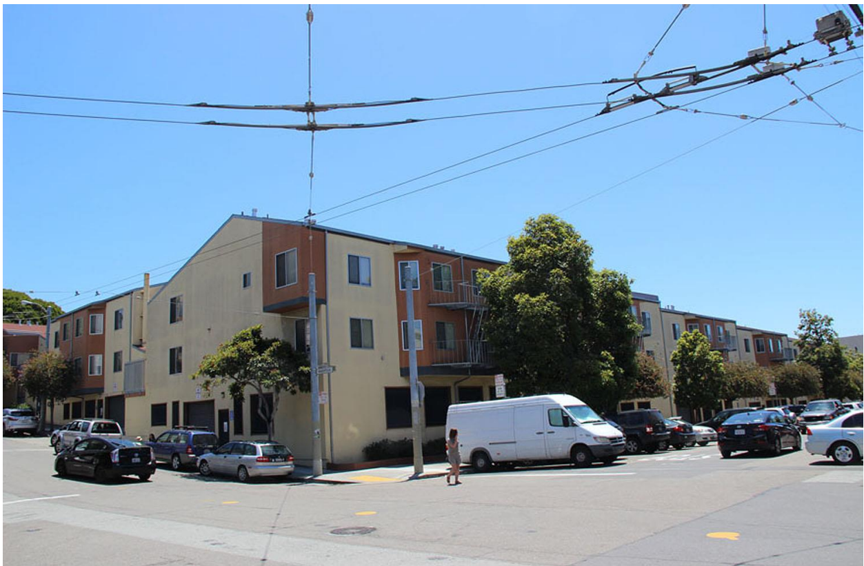
Figure 4. Mariposa Gardens, looking southeast from Mariposa and Hampshire Streets.
