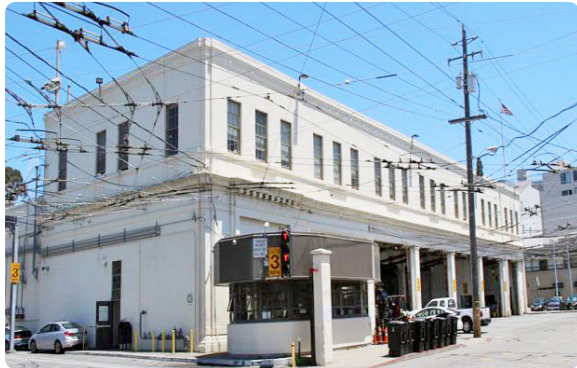
Image 1: View northeast of office wing primary façade along Mariposa Street.
