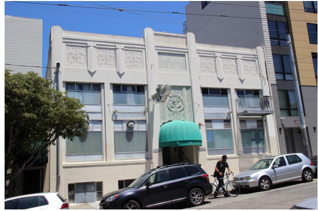
Figure 3. Verdi Club, 2440 Mariposa Street.
