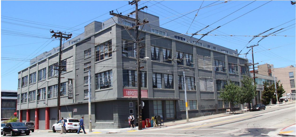
Figure 9. Former Best Foods Extension at 1890 Bryant Street, looking northwest.
