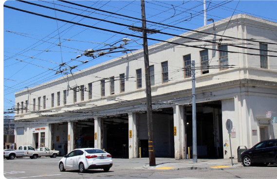
Image 2: View northwest of office wing primary façade along Mariposa Street (left), and secondary façade along Hampshire Street (right).
