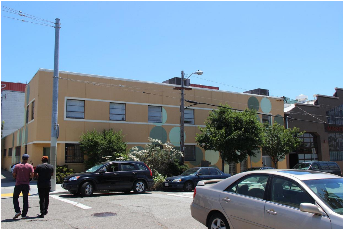
Figure 6. 501 York Street, looking southeast.
