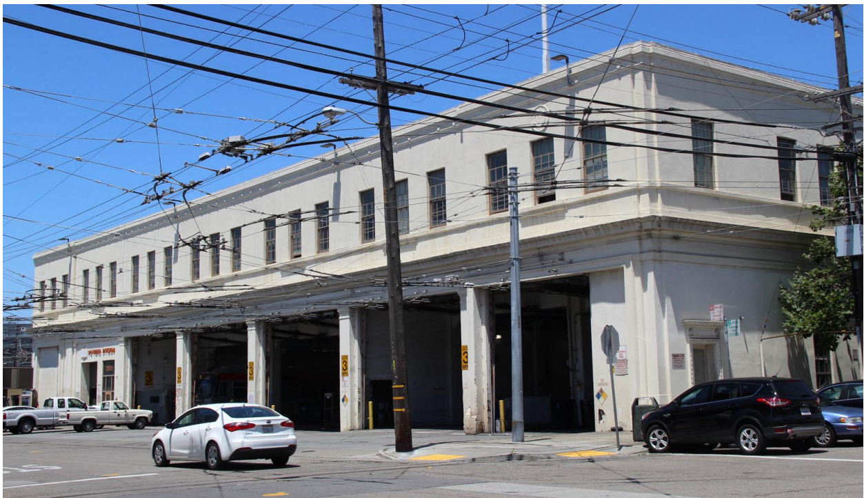
Figure 34. Primary façade of maintenance/operations building, looking northwest from Hampshire and Mariposa Streets.
