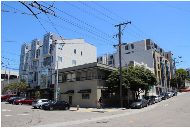
Figure 2. 2440 Mariposa Street (foreground).
