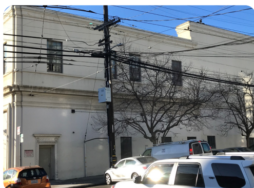
Image 7: Detail view of office wing secondary façade. Note character-defining features including molded concrete and cement plaster ornament, reentrant corner detailing, double-hung metal windows, and pedestrian door surround.
