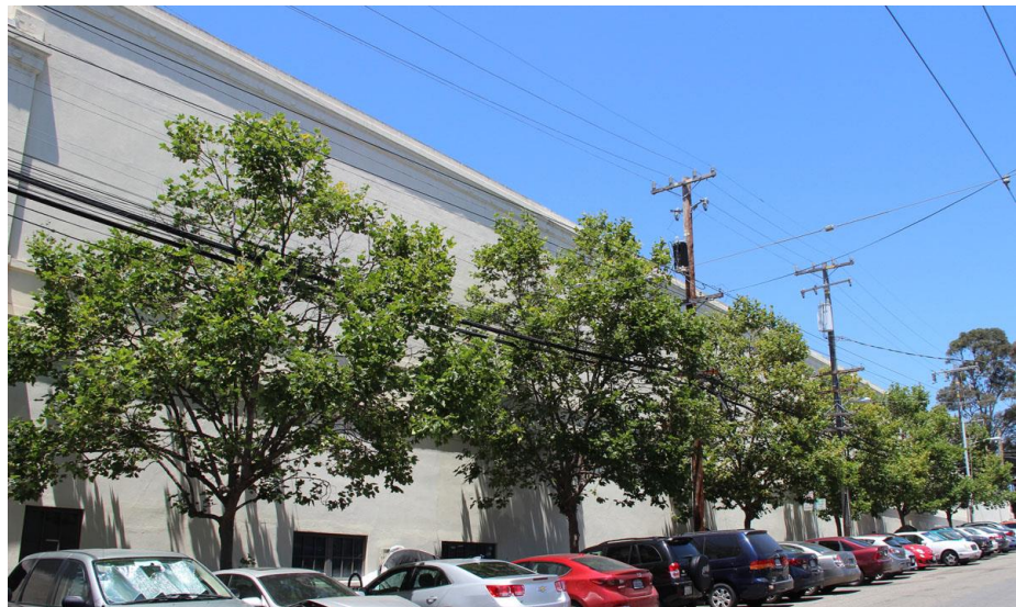
Figure 42. Middle section of secondary façade, looking northwest.
