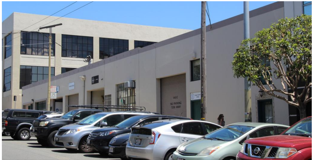
Figure 21. 445 Hampshire Street, looking northeast.
