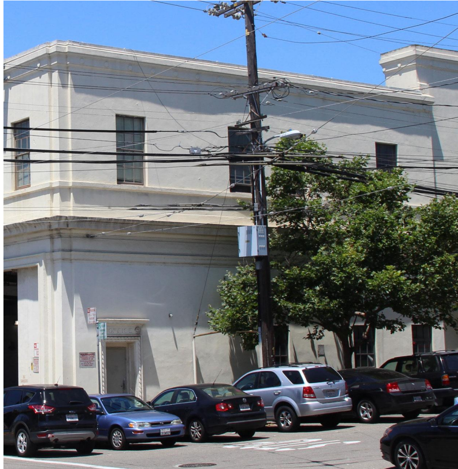
Figure 41. Southernmost section of secondary façade facing Hampshire Street, looking northwest.
