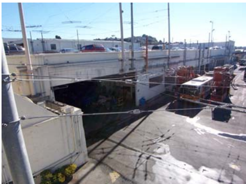
100_5696.JPG, 11/20/2007, view to E
