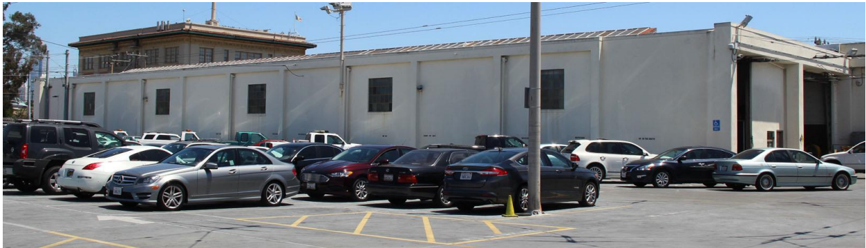
Figure 48. West façade of second floor maintenance shops, looking northeast from parking deck.
