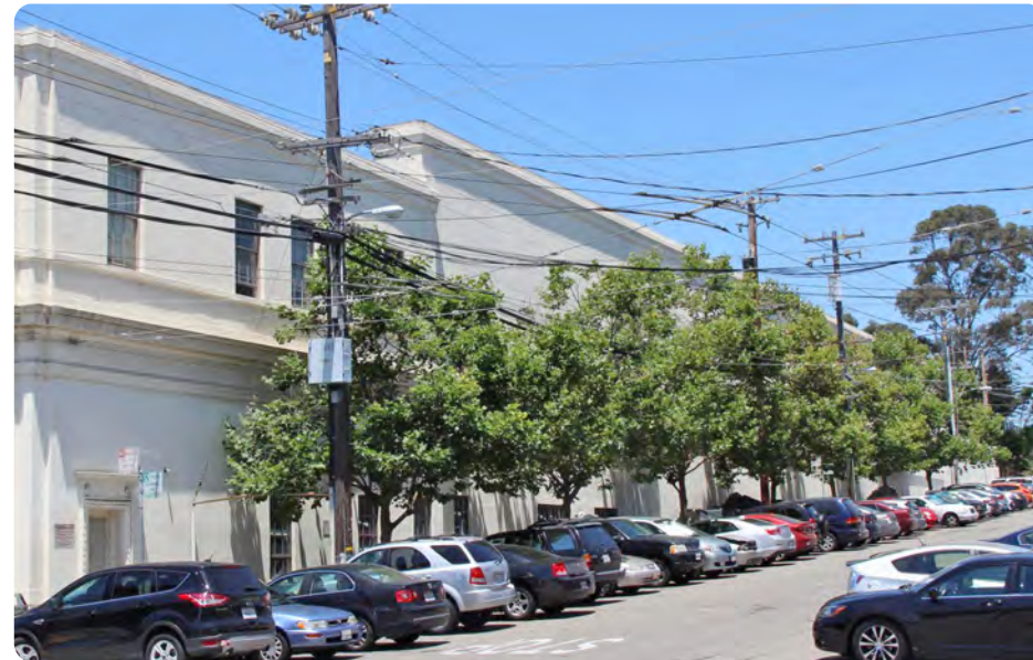
View B: Hampshire Street Looking North, Existing
