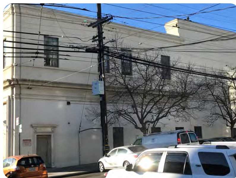
Image 7: Detail view of office wing secondary façade. Note character-defining features including molded concrete and cement plaster ornament, reentrant corner detailing, double-hung metal windows, and pedestrian door surround.
