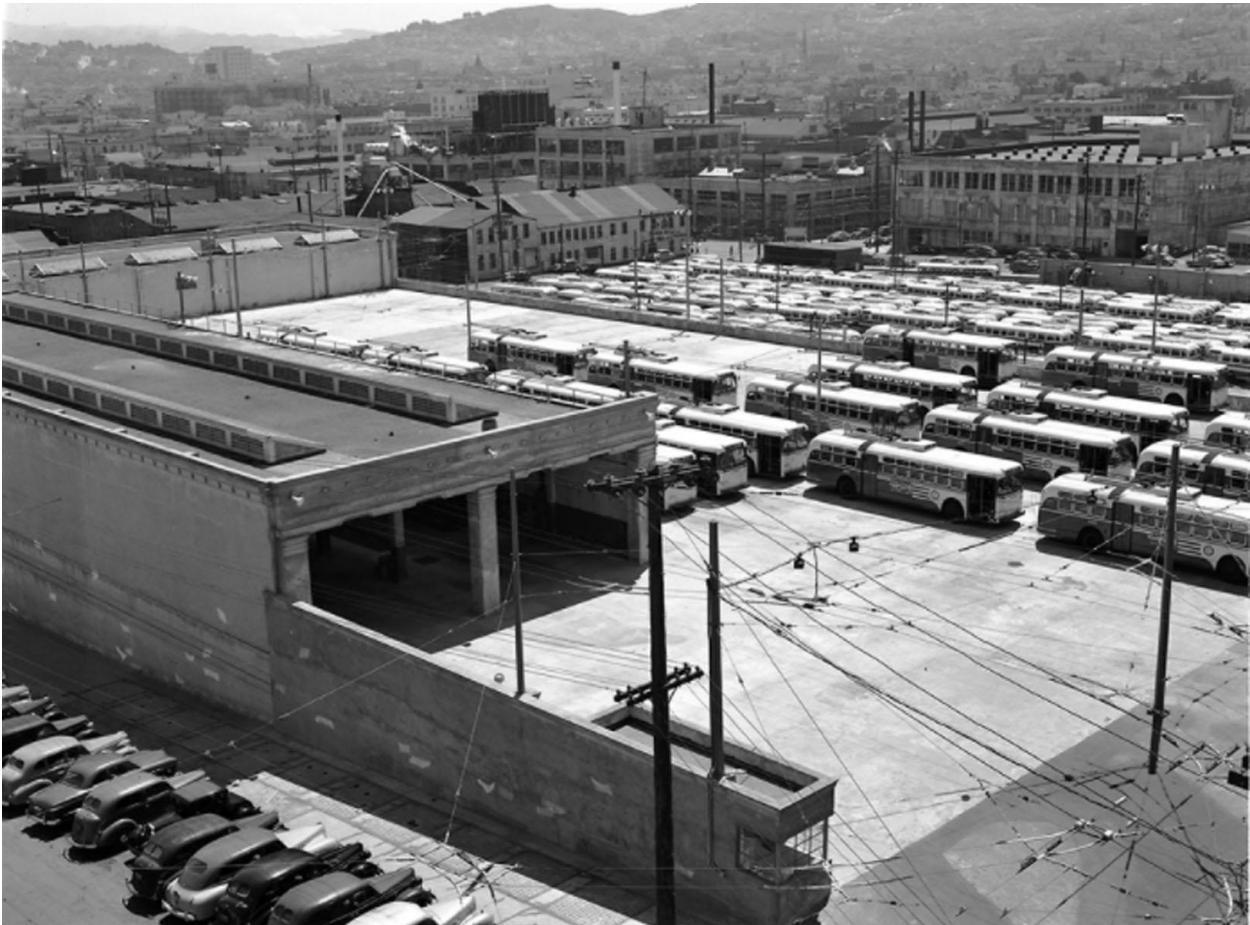
Figure 82. Appearance of the Potrero Trolley Coach Division Facility following 1949 remodel. Source: SFMTA Photography Department and Archive, Image No. X2104
