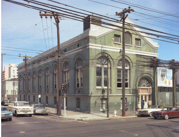
Figure 90. Turk and Fillmore Substation, 1966; built 1895. Source: SFMTA Photography Department and Archive, Image No. X9762_1
