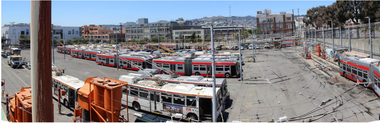
Figure 22. Mariposa Bus Yard, looking southwest.
