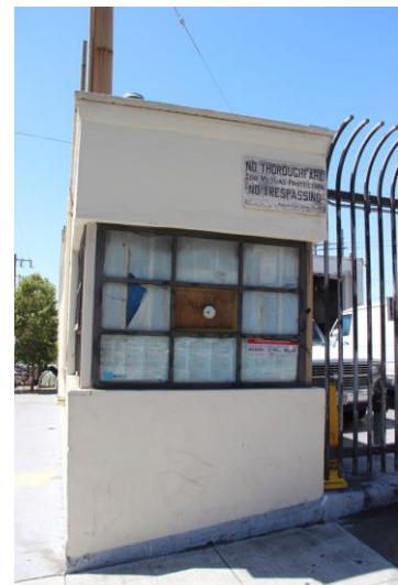
Figure 44. North wall of former control room
