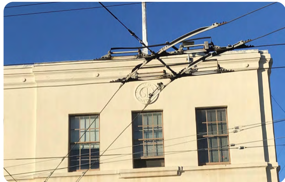
Image 6: Detail view of office wing primary façade. Note character defining features including molded concrete and cement plaster ornament, fenestration pattern of groups of three double-hung metal windows, medallion featuring original Muni logo, and flagpole
