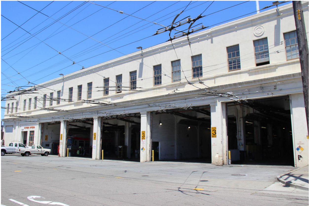
Figure 36. Primary façade, looking northwest.
