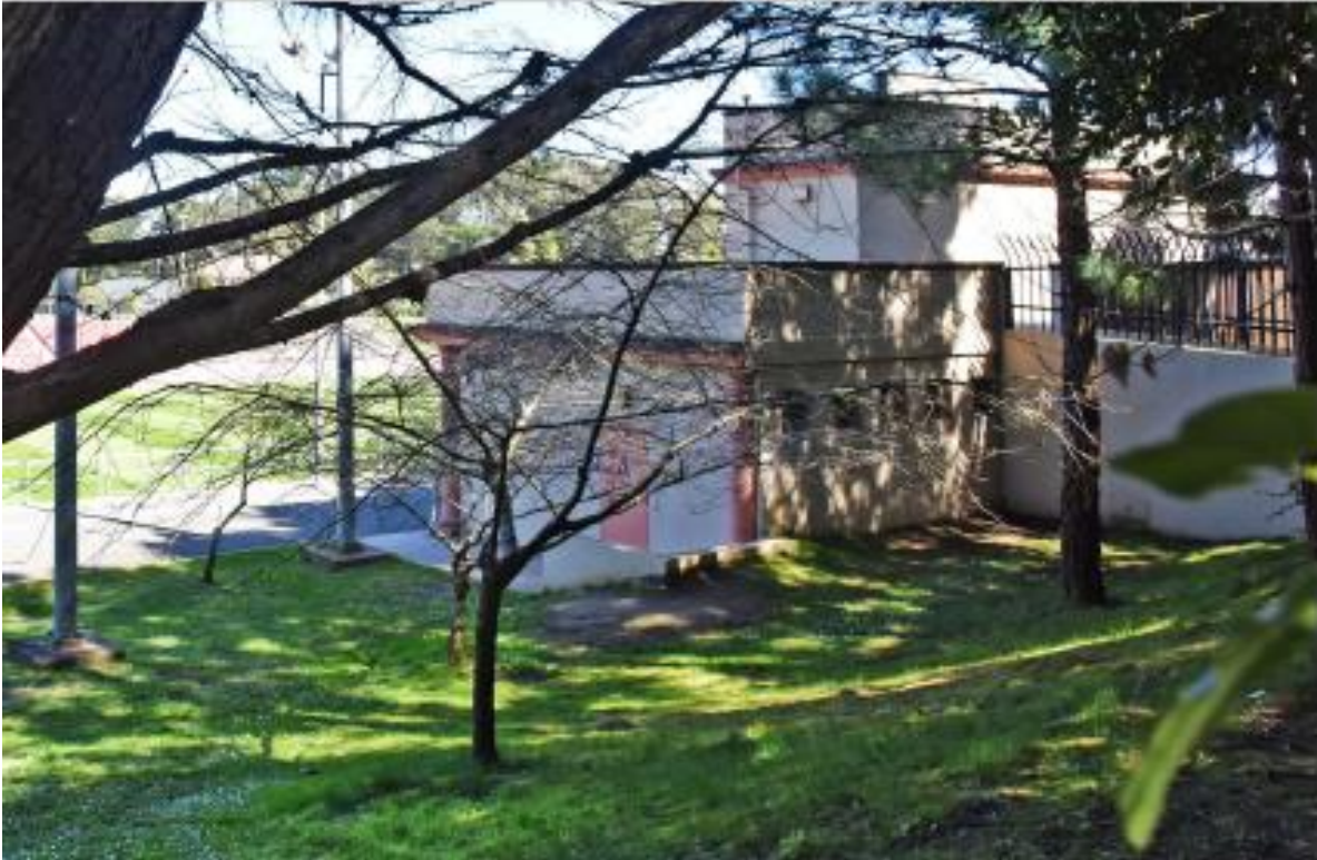
Above: South building, as seen from Frederick Street.
