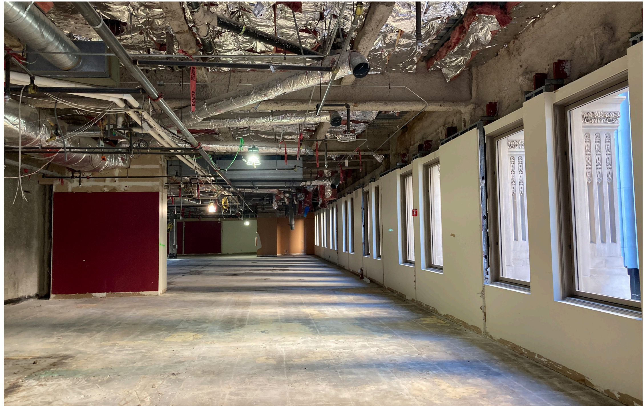
in-progress demolition at level 2 - space opened up and concrete structure exposed
