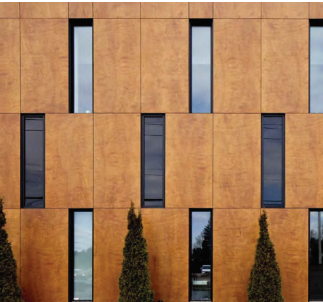
03 WOOD TEXTURE RAIN SCREEN EXTERIOR CLADDING SYSTEM & WINDOW SHADE
