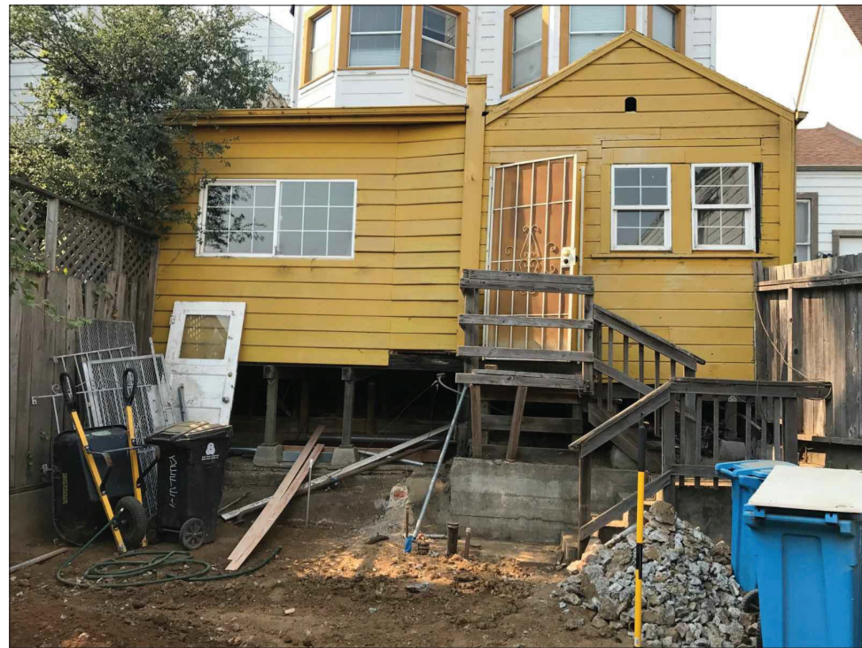
PRIOR TO DEMOLITION PICTURES
