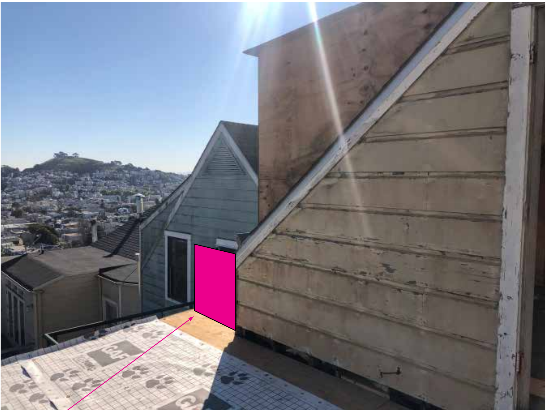
42" high solid wing wall between 486 and 480 Duncan.
