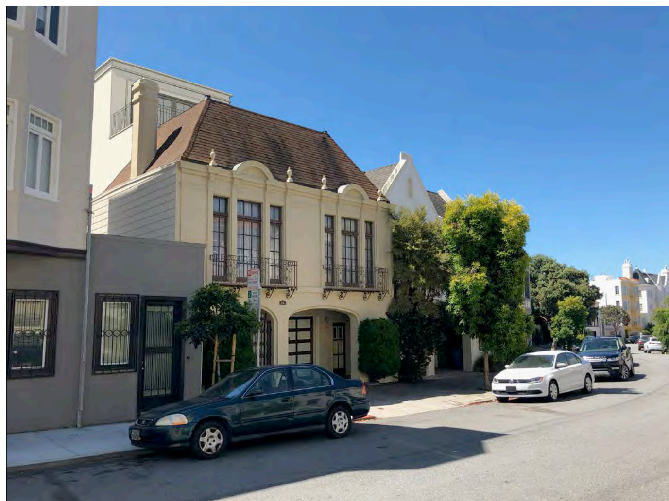
1 - METAL GUARDRAIL ON ROOF DECK
