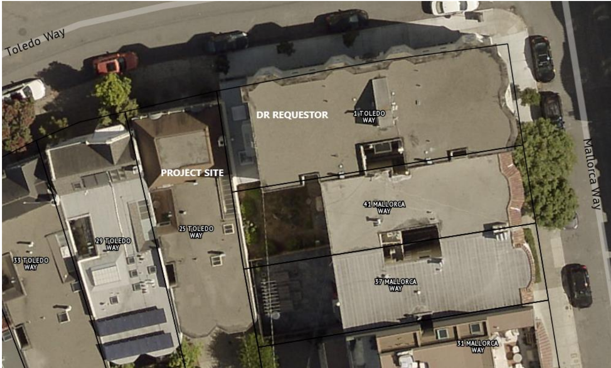
Figure 1. 25 Toledo is adjacent to and east of the 1 Toledo Apartment Building
