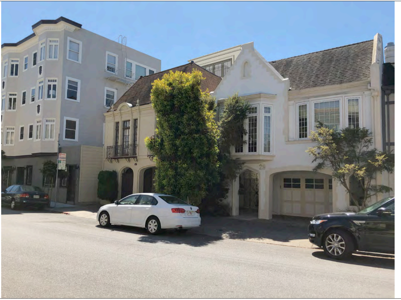
2 - METAL GUARDRAIL ON ROOF DECK
