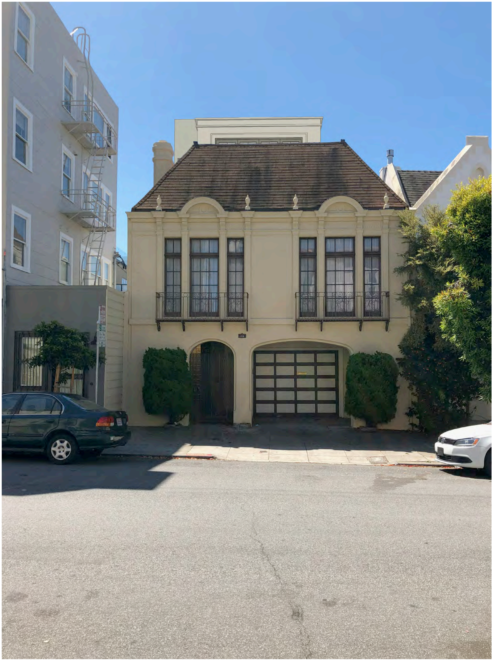
5 - GUARDRAIL ON ROOF DECK NOT VISIBLE
