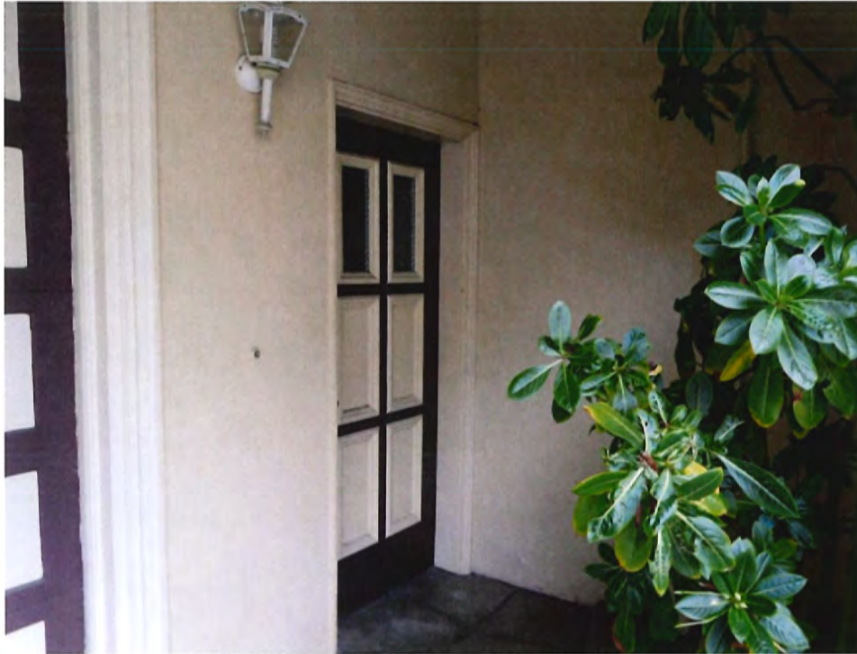
Pedestrian door near garage
