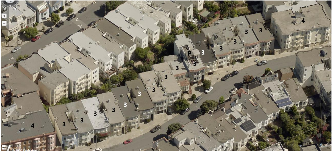
Figure 3. North block face of Toledo Way showing mid-block buildings are 3 stories (with two containing small pent rooms) with taller buildings on corners
