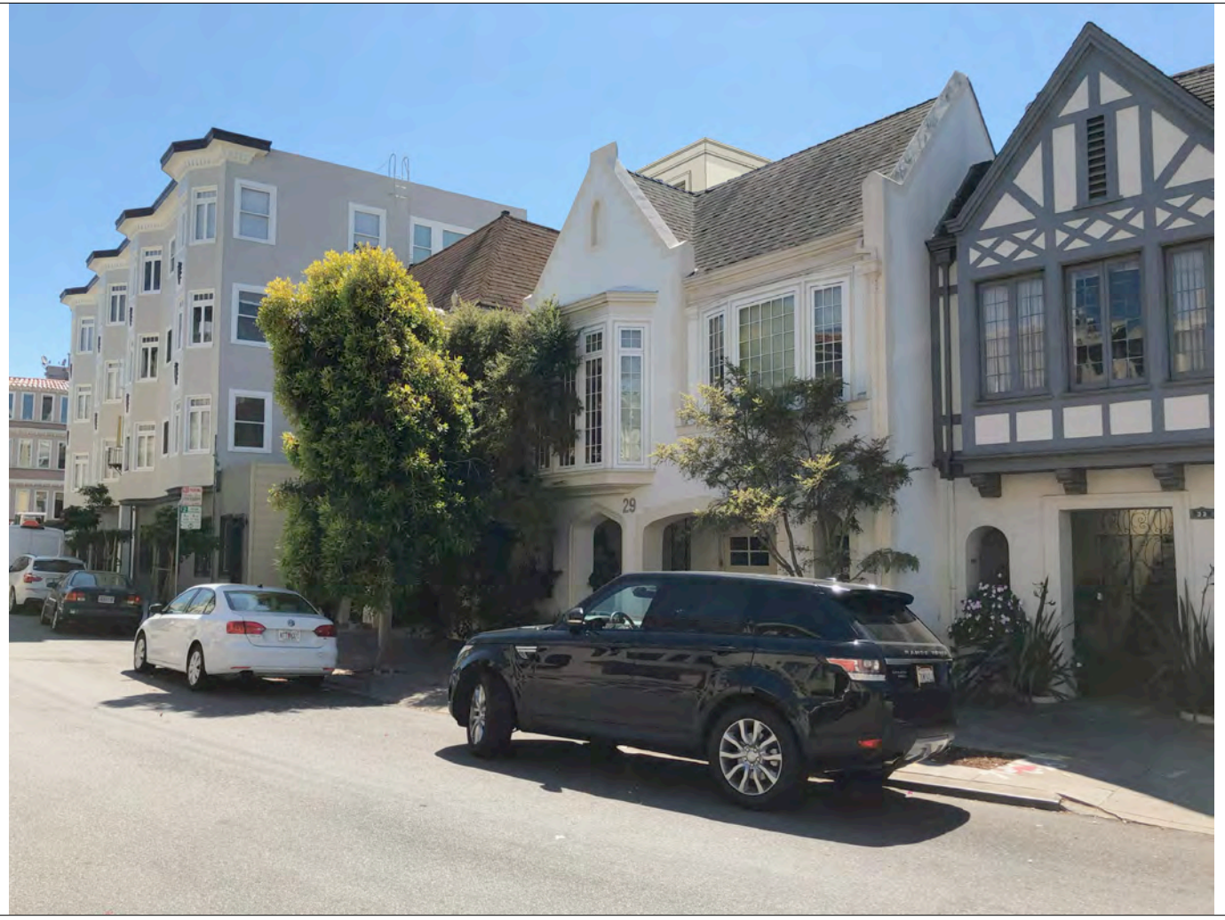
3 - GUARDRAIL ON ROOF DECK NOT VISIBLE
