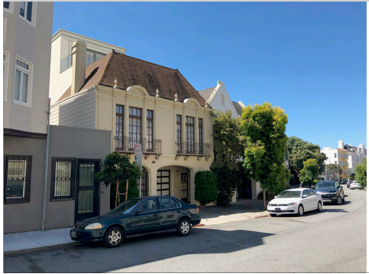
1 - GLASS GUARDRAIL ON ROOF DECK
