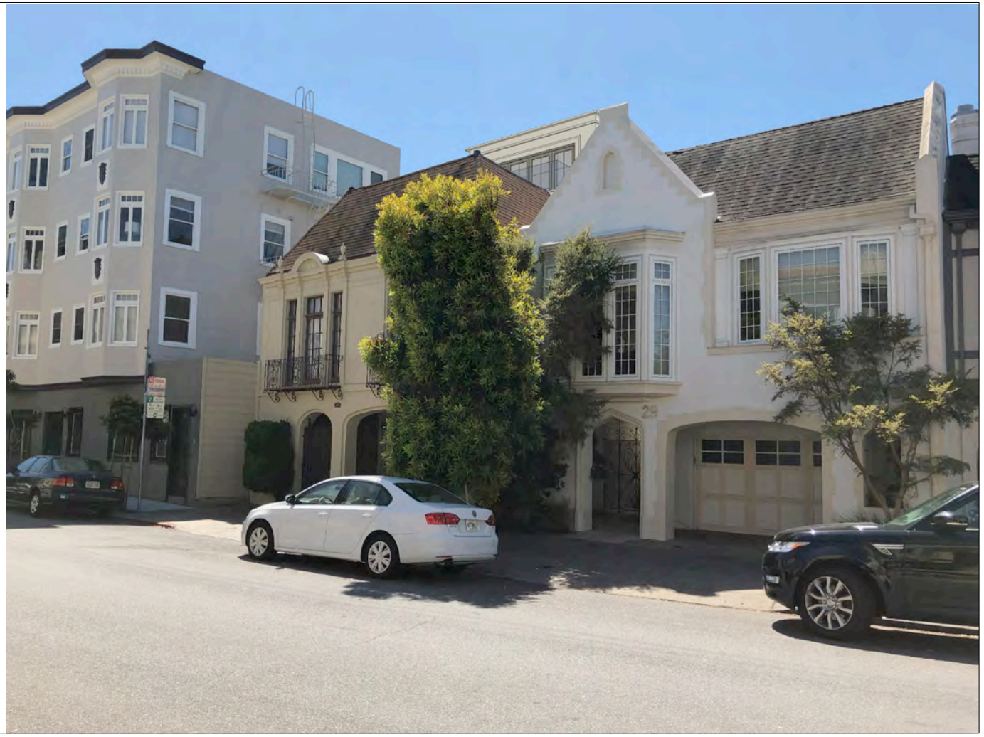
2 - GLASS GUARDRAIL ON ROOF DECK
