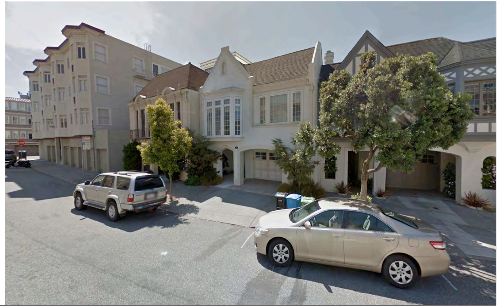
4 - GUARDRAIL ON ROOF DECK NOT VISIBLE
