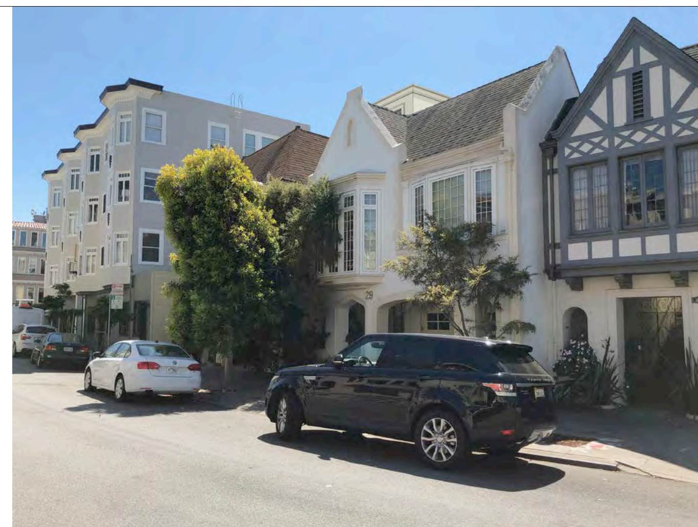
3 - GUARDRAIL ON ROOF DECK NOT VISIBLE
