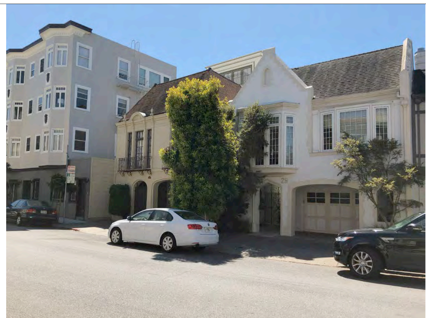
2 - METAL GUARDRAIL ON ROOF DECK
