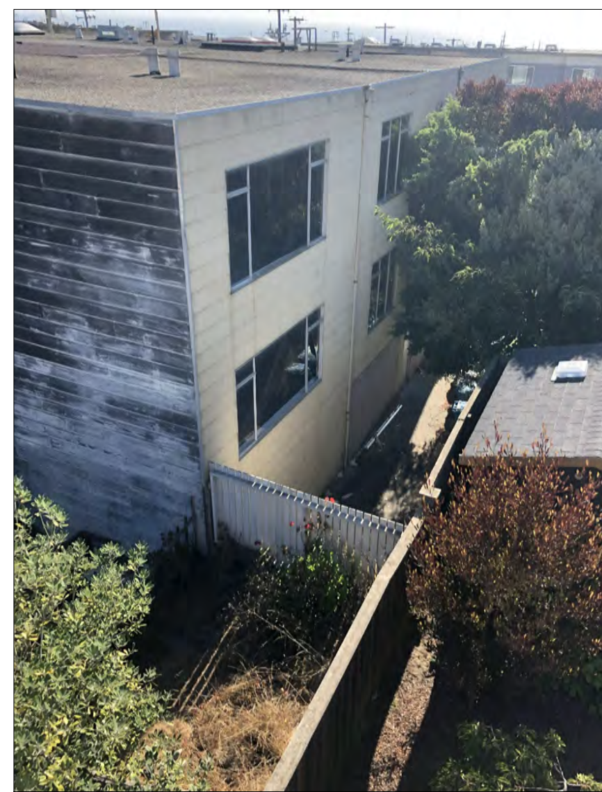
4 (E) REAR FACADE OF THE SUBJECT BUILDING N.T.S.
