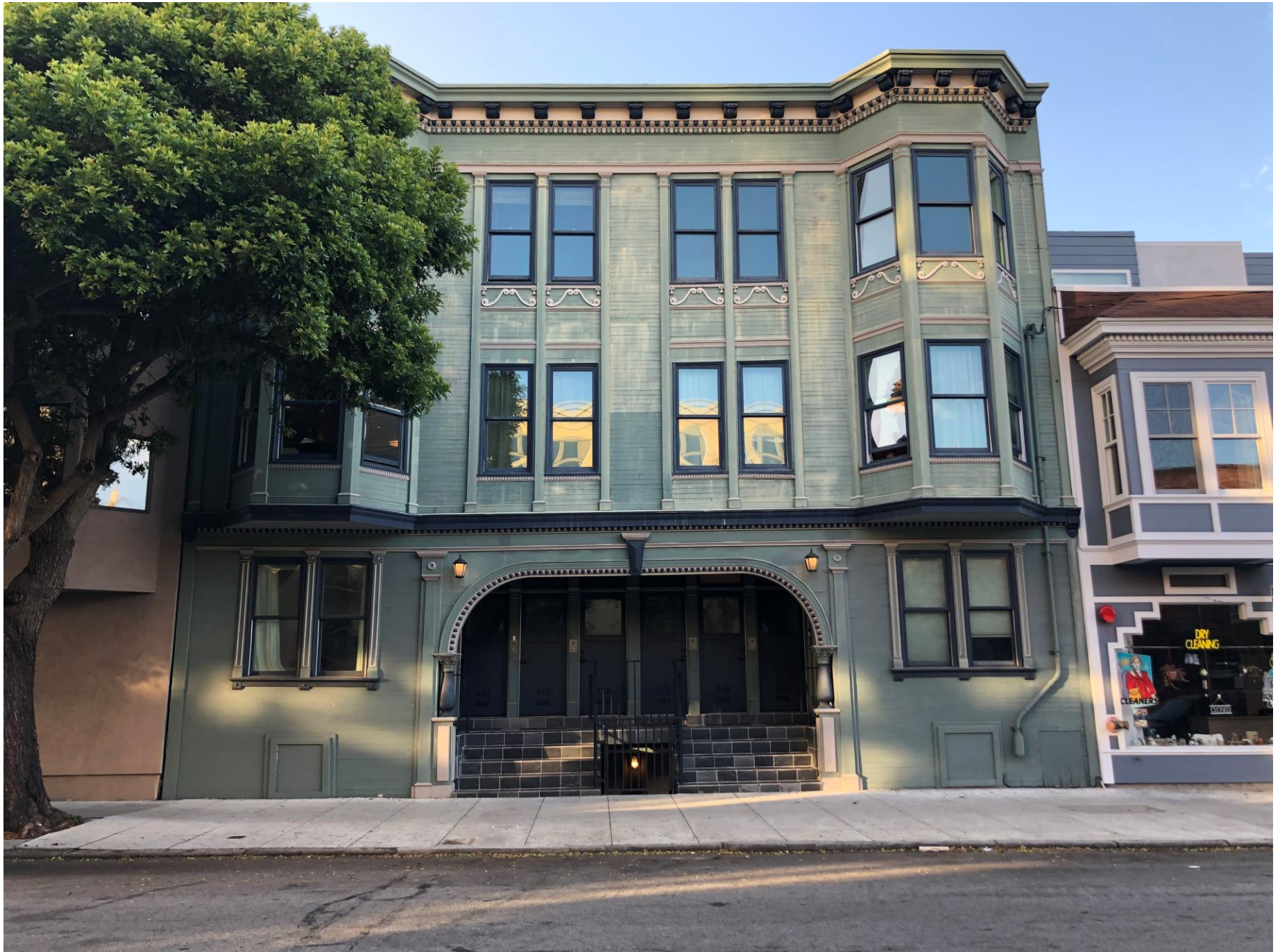
Front of Building
