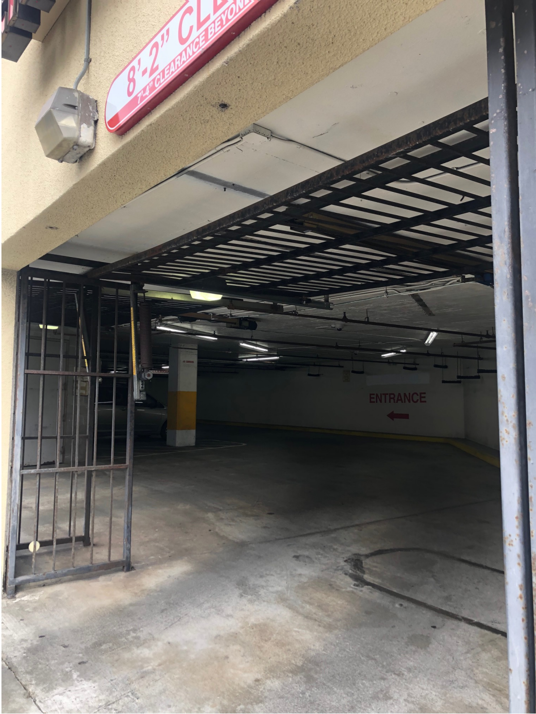
Close-up of parking structure entrance
