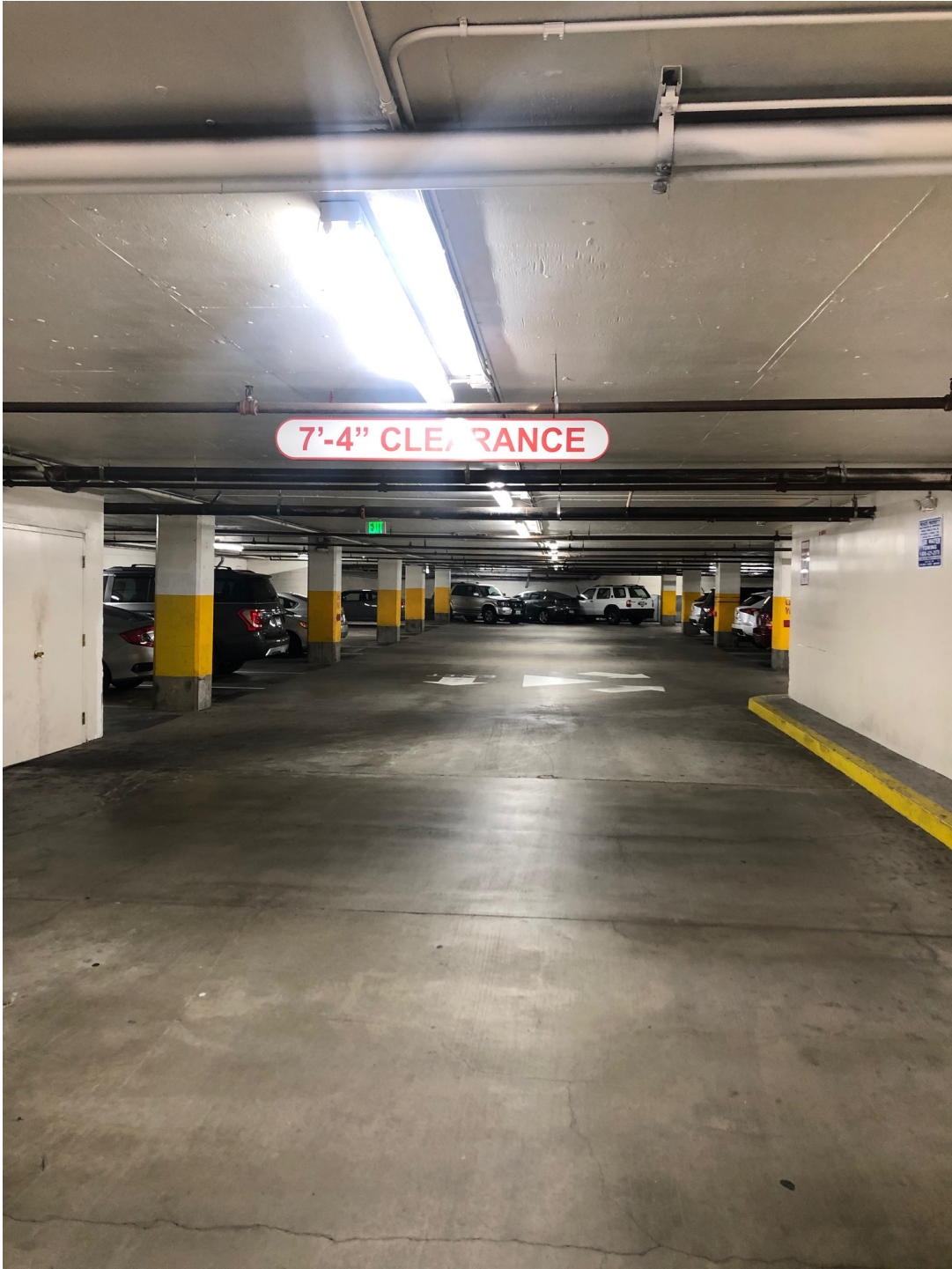
View of parking structure and 7'-4" internal Clearance Sign
