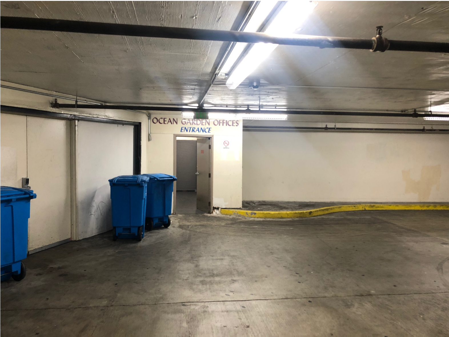
View of facility's internal entrance from parking structure
