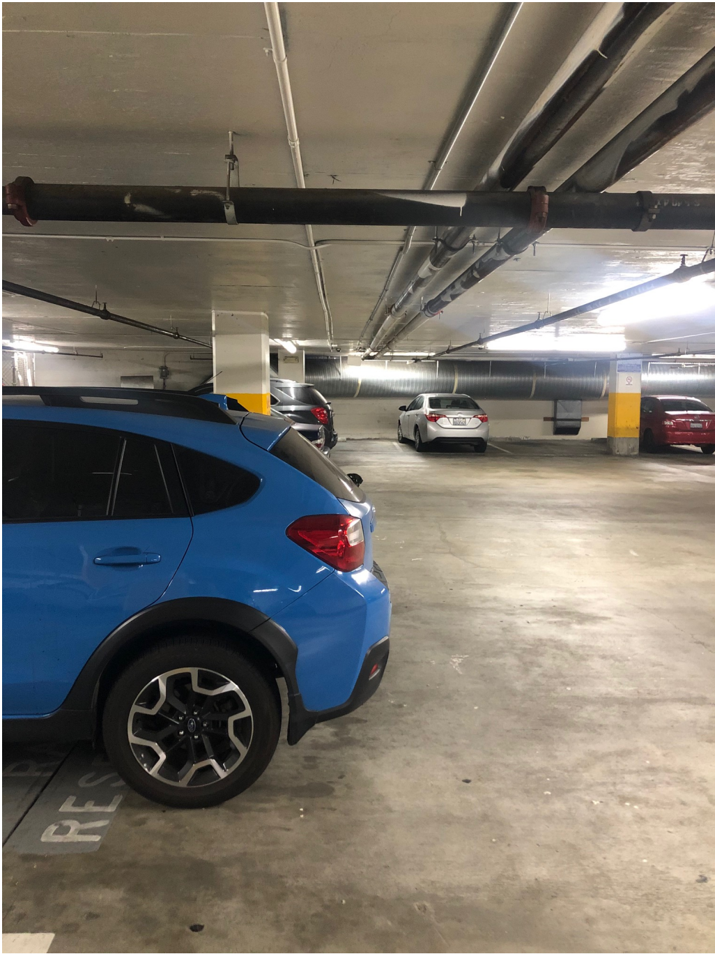
Internal view of parking structure
